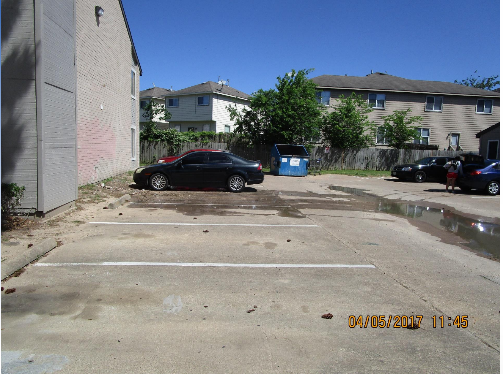
Sewage discharge flowing untreated to recreational waters.
