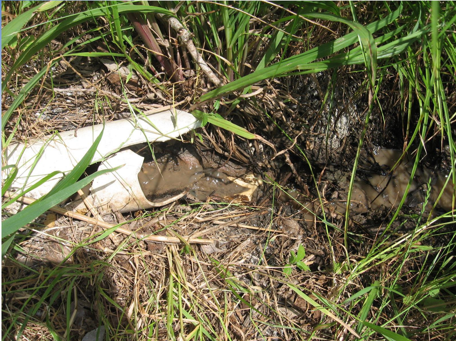
Discharge from sump at a construction vehicle washing area.
