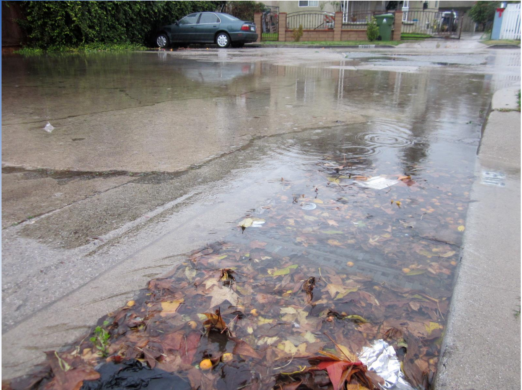
Leaves and debris causing street flooding.
