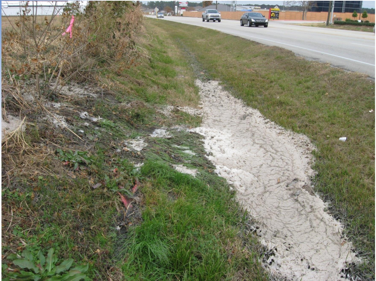
Utility company discharge of sewage to ditch.
