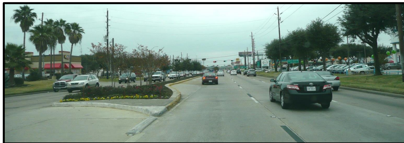
Figure 9. FM 1960 Intersection Turn Bay
