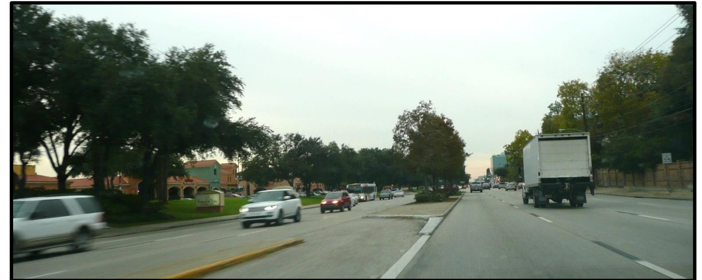
Figure 6. Example of Median Treatments on FM 1093 West of Gesner Left Turn Bay and Planter
