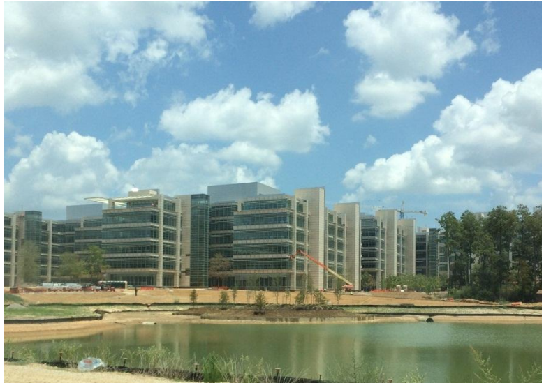
ExxonMobil campus under construction.
