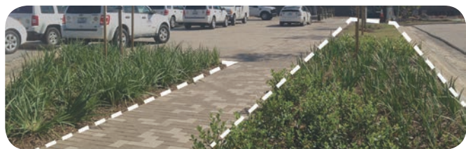
Bioswale, Houston Permitting Center
