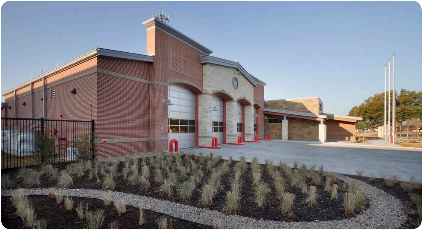
Native Plantings, Fire Station 90
