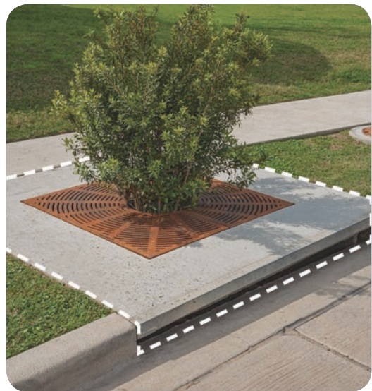
Stormwater Planter Box, Darling Street
