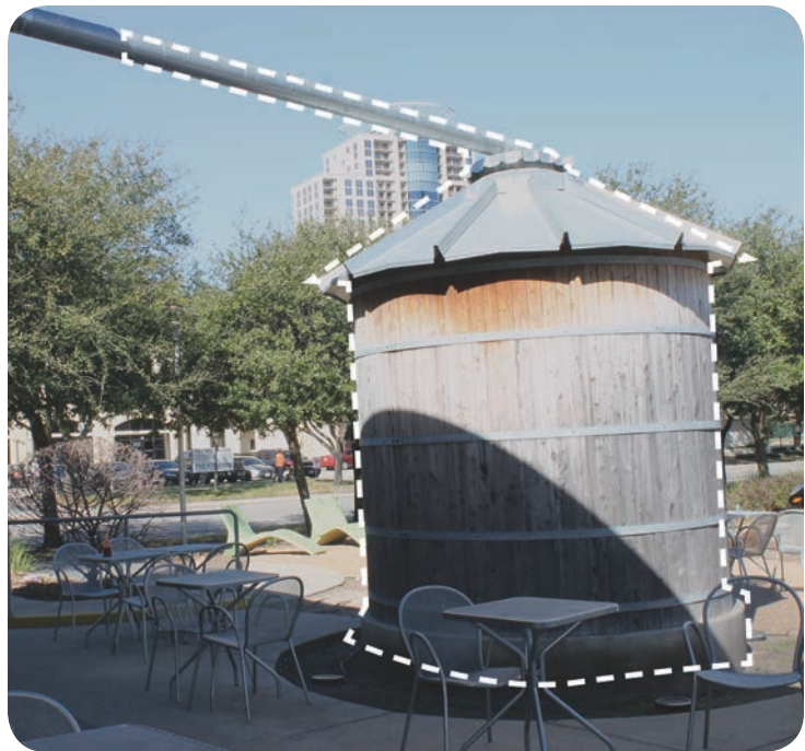
Cistern, Grocery Store in Houston
