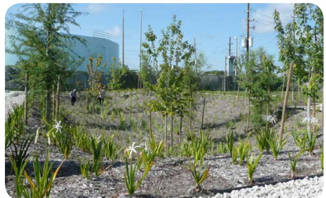
Rainwater Harvesting Cisterns and Rain Garden with Native Plantings, Fire Station 90
