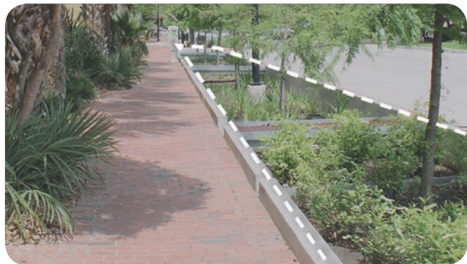
Bioswale, Bagby Street
