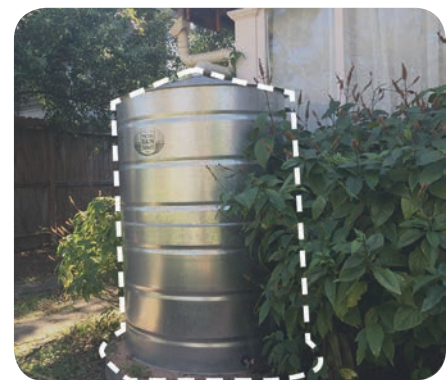
Rain Barrel, Residence in Houston
