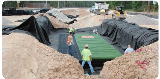
Bioswale and Underground Storage Construction, Birnamwood Drive
