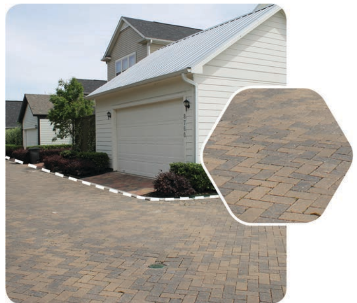
Permeable Pavement, Kempwood Manor
