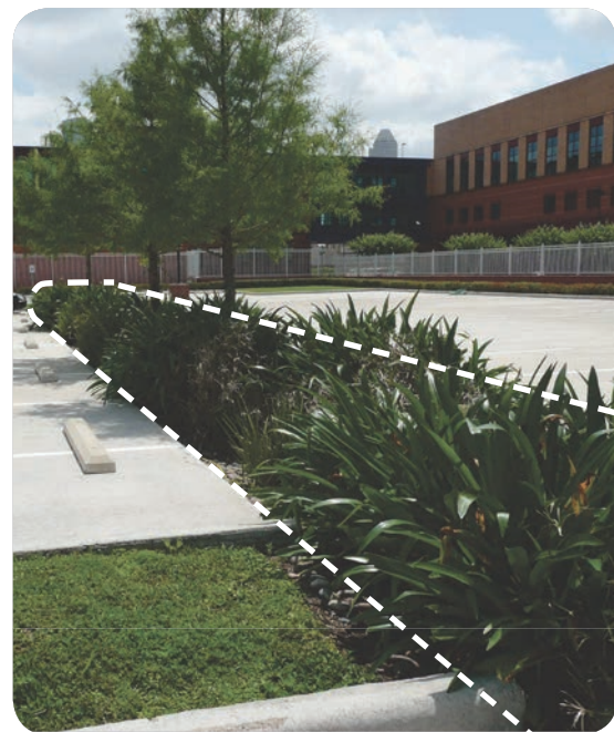
Vegetated Swale, Federal Reserve Bank
