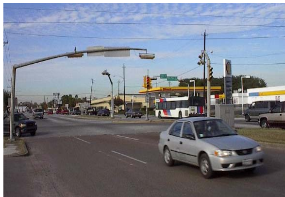
Traffic Along Existing SH 35 at Park Place/Long Drive
