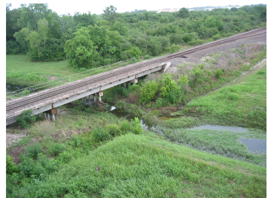
BNSF RR Bridge Over Clear Creek
