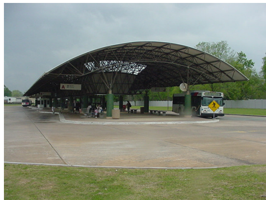
Southeast METRO Transit Center
