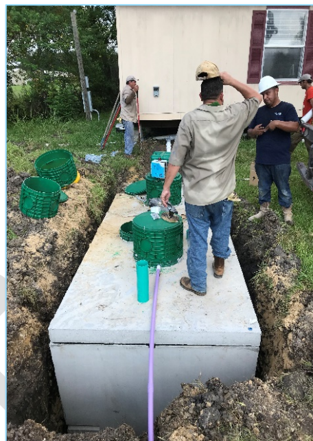
Figure 4. Septic tank replacement
