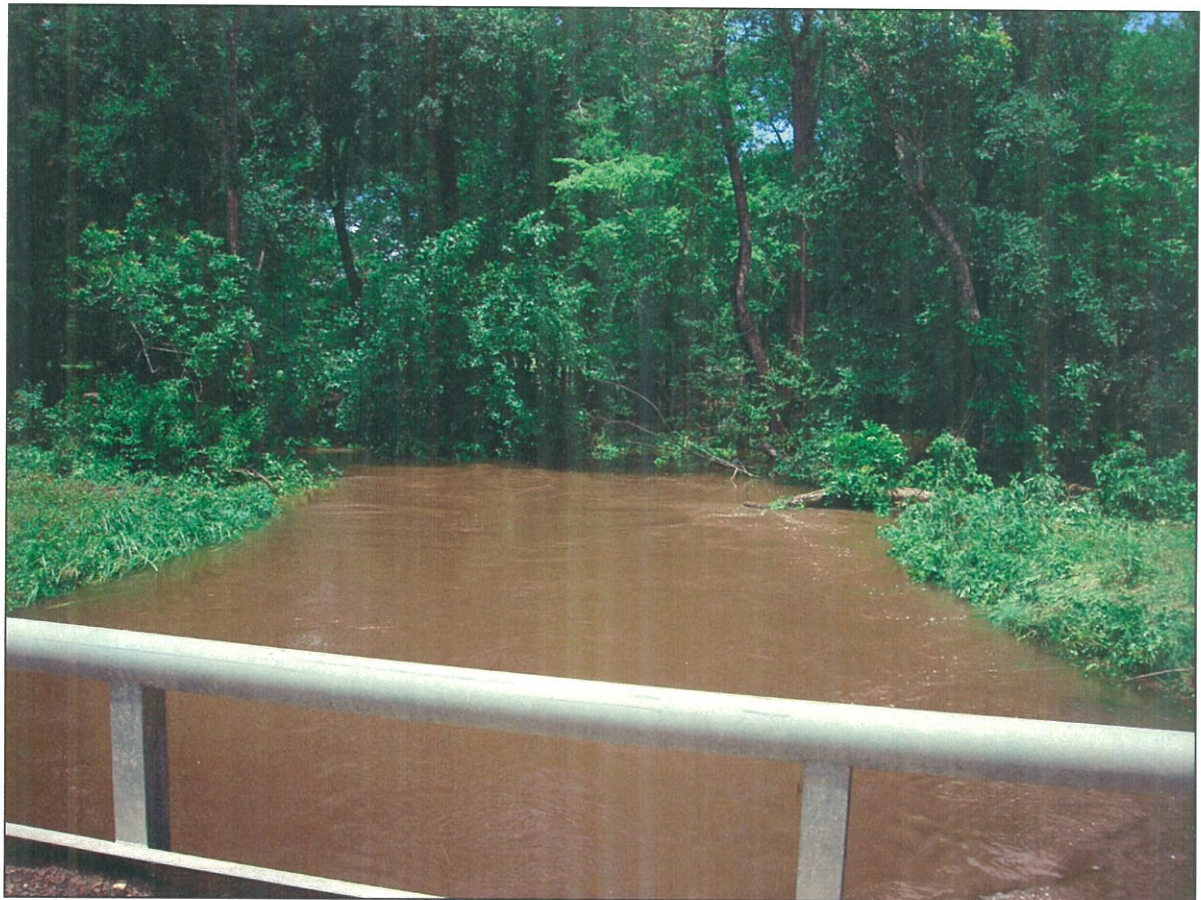
West Fork Mill Creek at Industry Rd looking upstream 5.28.07
