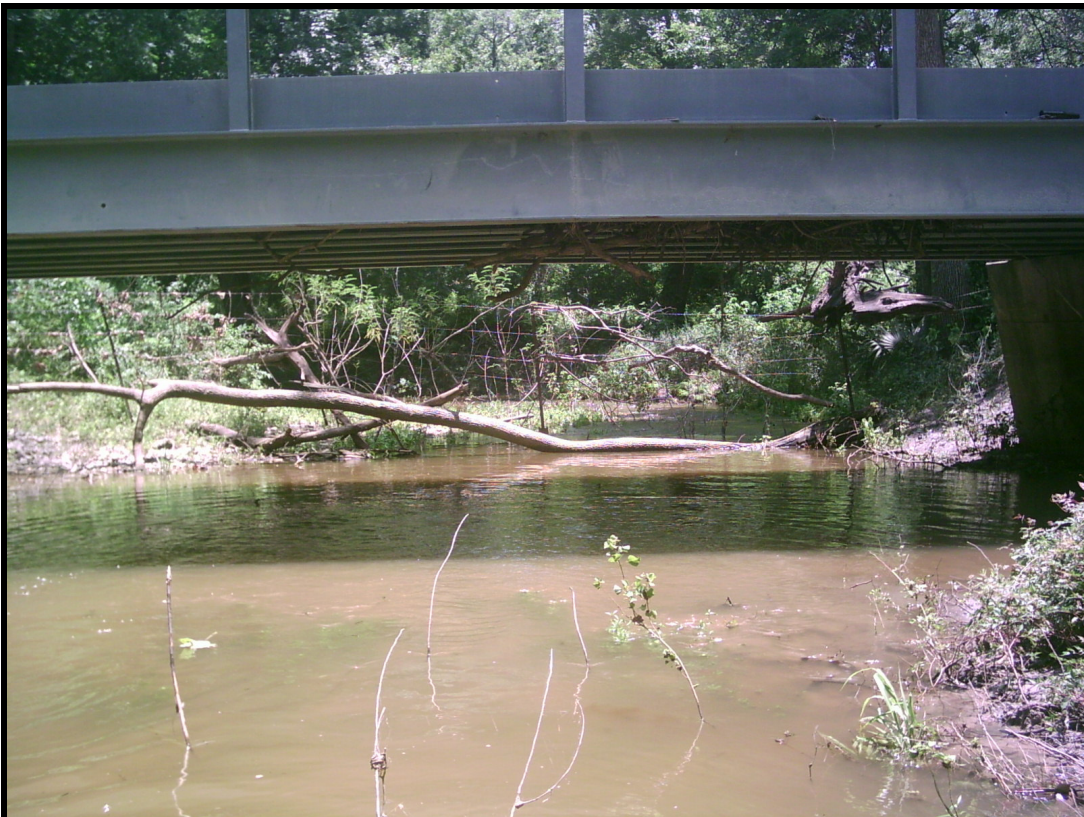
UAA1 (West Fork): Transect 1, facing downstream.
