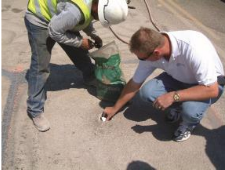
FIGURE 4-7 WIRELESS MAGNETOMETER BEING INSTALLED FOR MOTORIZED TRAFFIC
