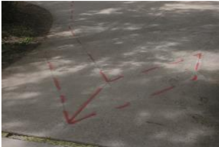
FIGURE 4-3D EXAMPLES OF INDUCTANCE LOOP DETECTOR SHAPES FOR BICYCLIST COUNTING DOUBLE CHEVRON SHAPE; PHOTO
