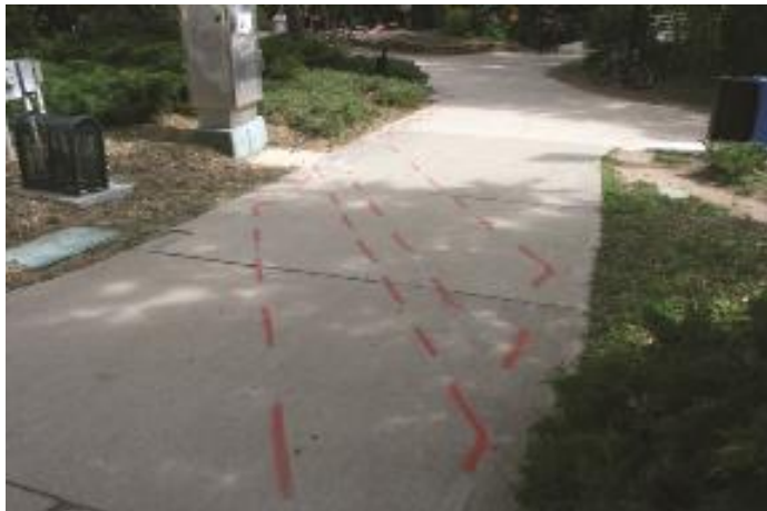
FIGURE 4-3F EXAMPLES OF INDUCTANCE LOOP DETECTOR SHAPES FOR BICYCLIST COUNTING ALTERNATIVE DOUBLE CHEVRON SHAPE; PHOTO
