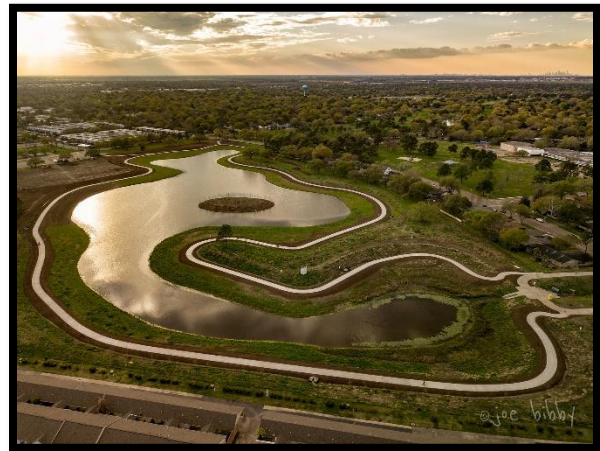
Figure 5. Aerial photo of one of the basins at EG.
