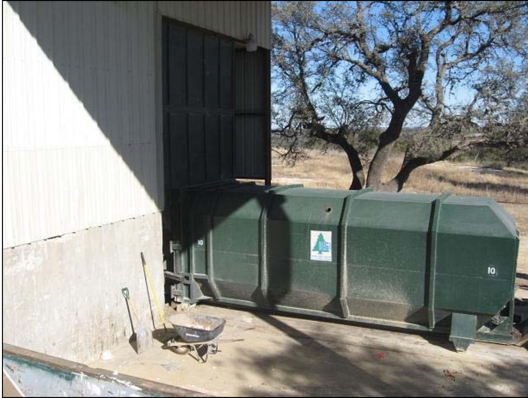
Figure 3-3. Compactor Receiving Unit
