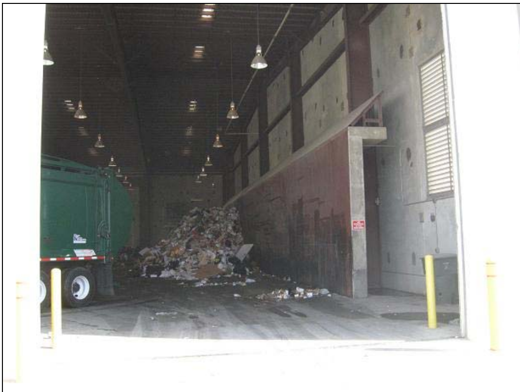
Figure 4-8. Structural Push Wall on South End of Tipping Floor
