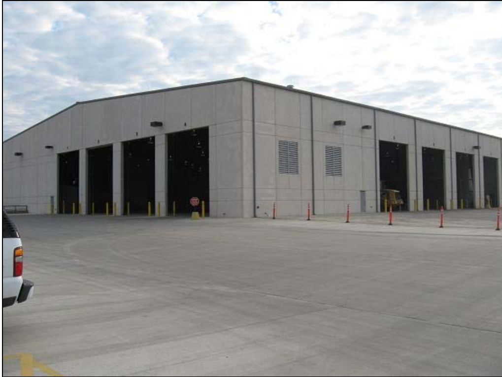
Figure 4-1. Transfer Station Building
