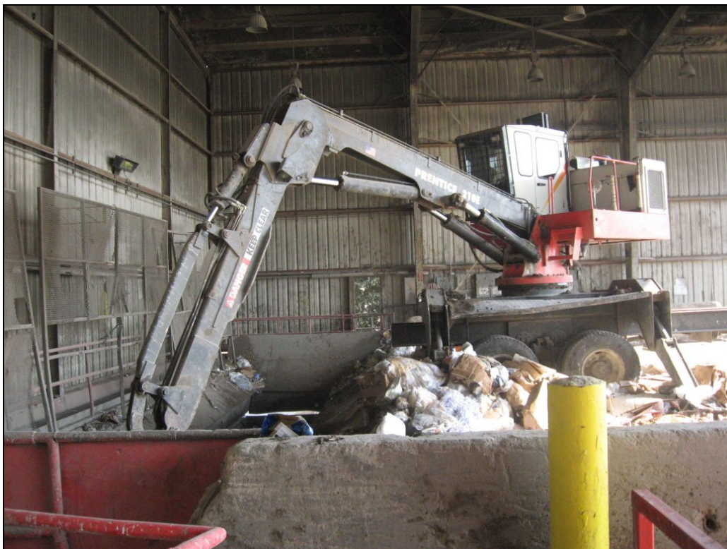
Figure 2-4. Crane Compacting and Managing Waste in Open Top Trailer
