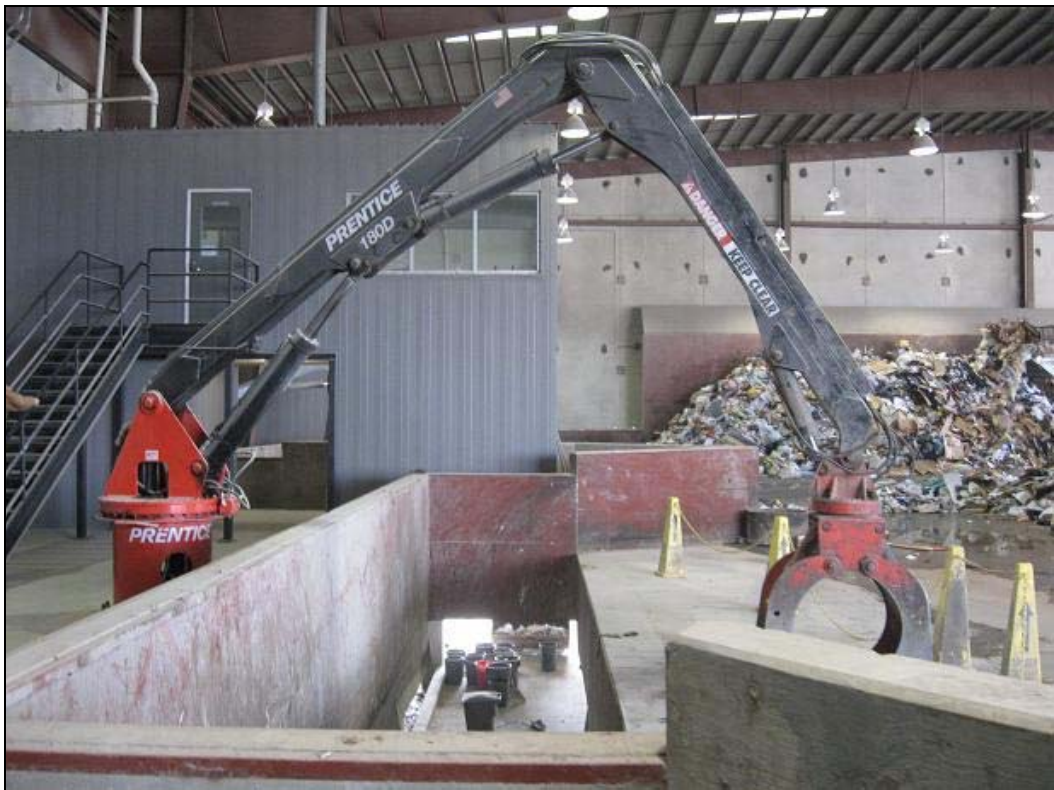
Figure 4-4. Stationary Crane Loading Transfer Trailer
