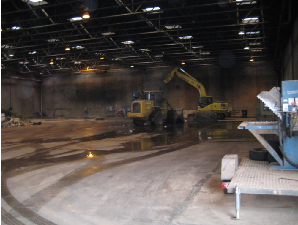
Figure 1-5. Transfer Station Floor
