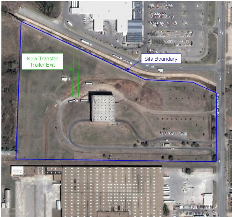
Figure 1-1. Site Aerial (Source: Google Earth)
