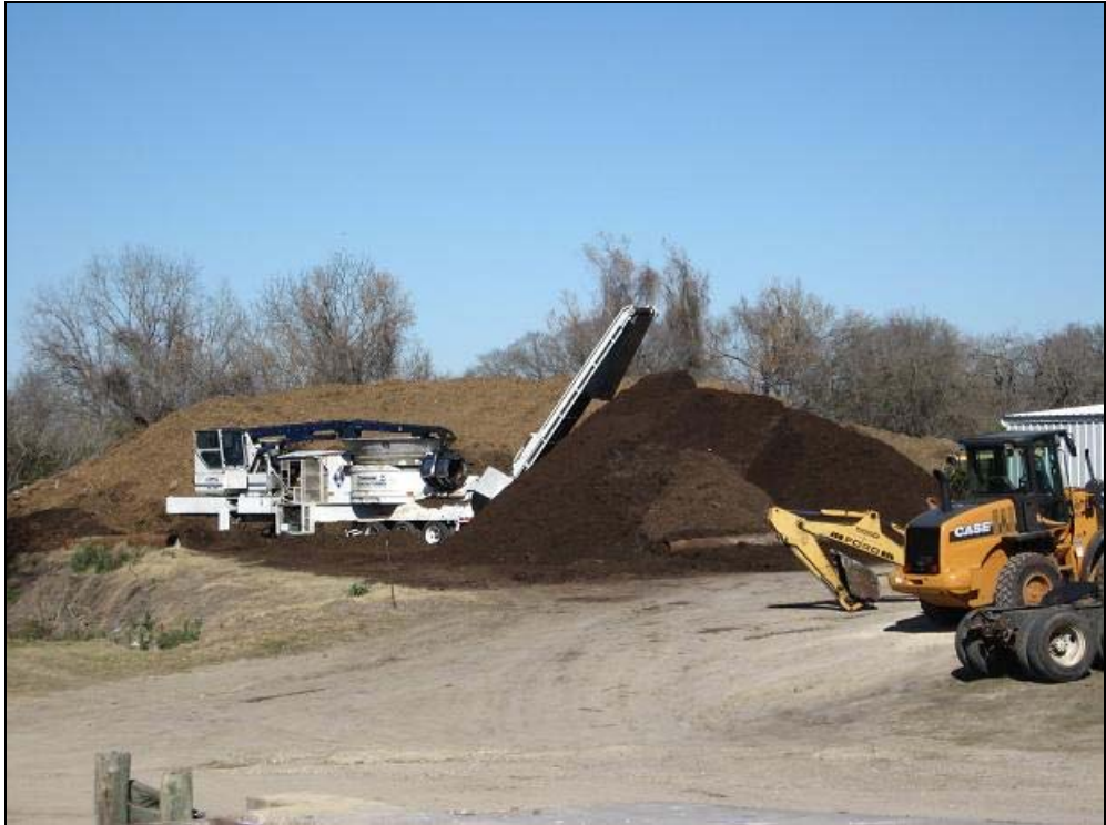
Figure 4-6. Mulching Operation Adjacent to Transfer Station
