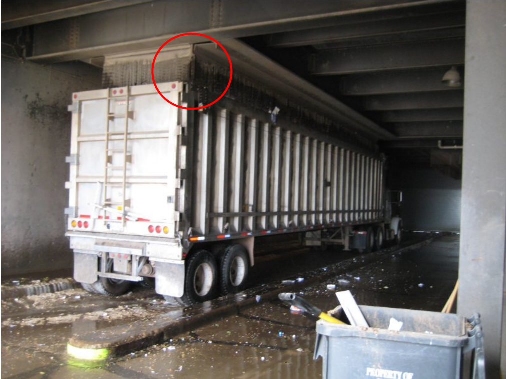
Figure 1-7. Transfer Trailer Being Loaded (chain curtain identified in picture)
