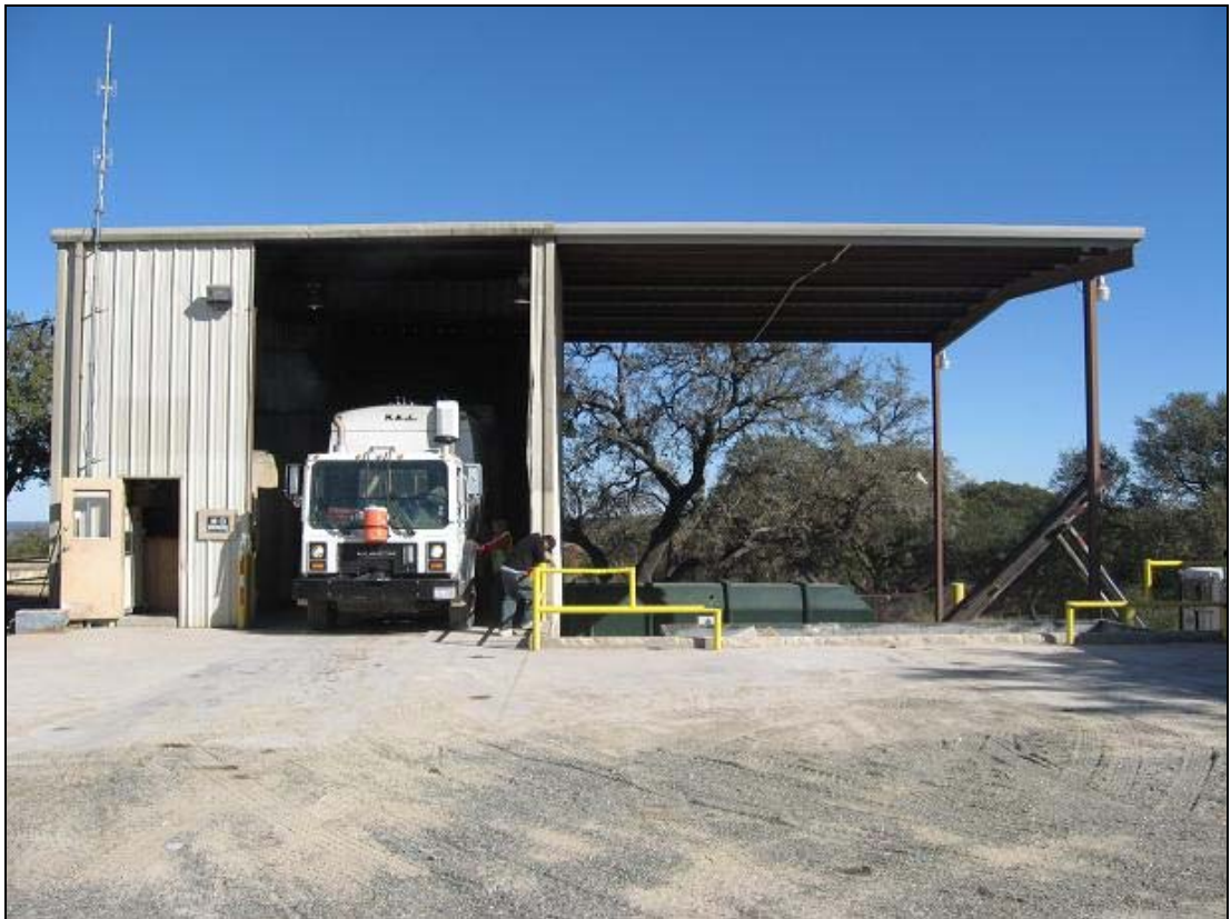
Figure 3-2. Collection Vehicle Direct Dumping into Compactor
