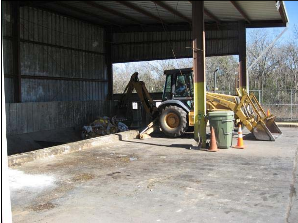
Figure 4-3. Wheeled Loader/Backhoe Compacting Waste
