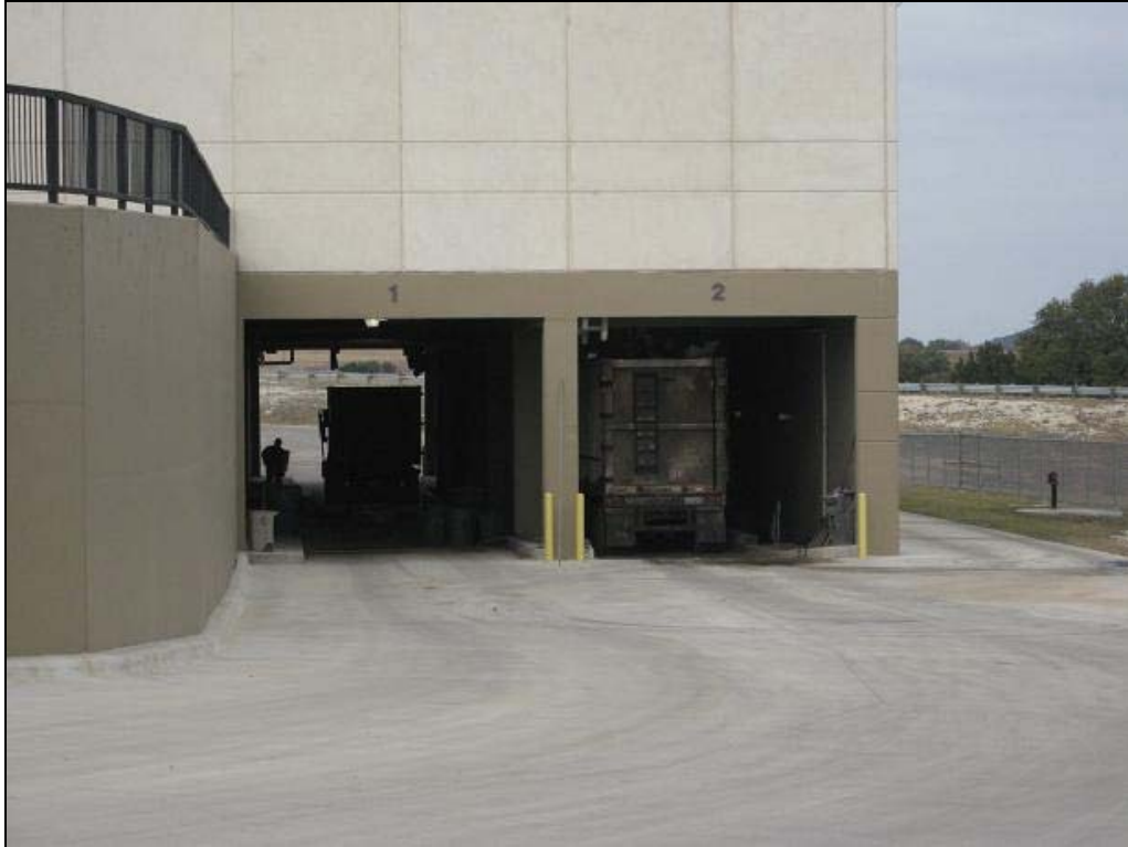
Figure 4-7. Below Grade Tunnel for Transfers
