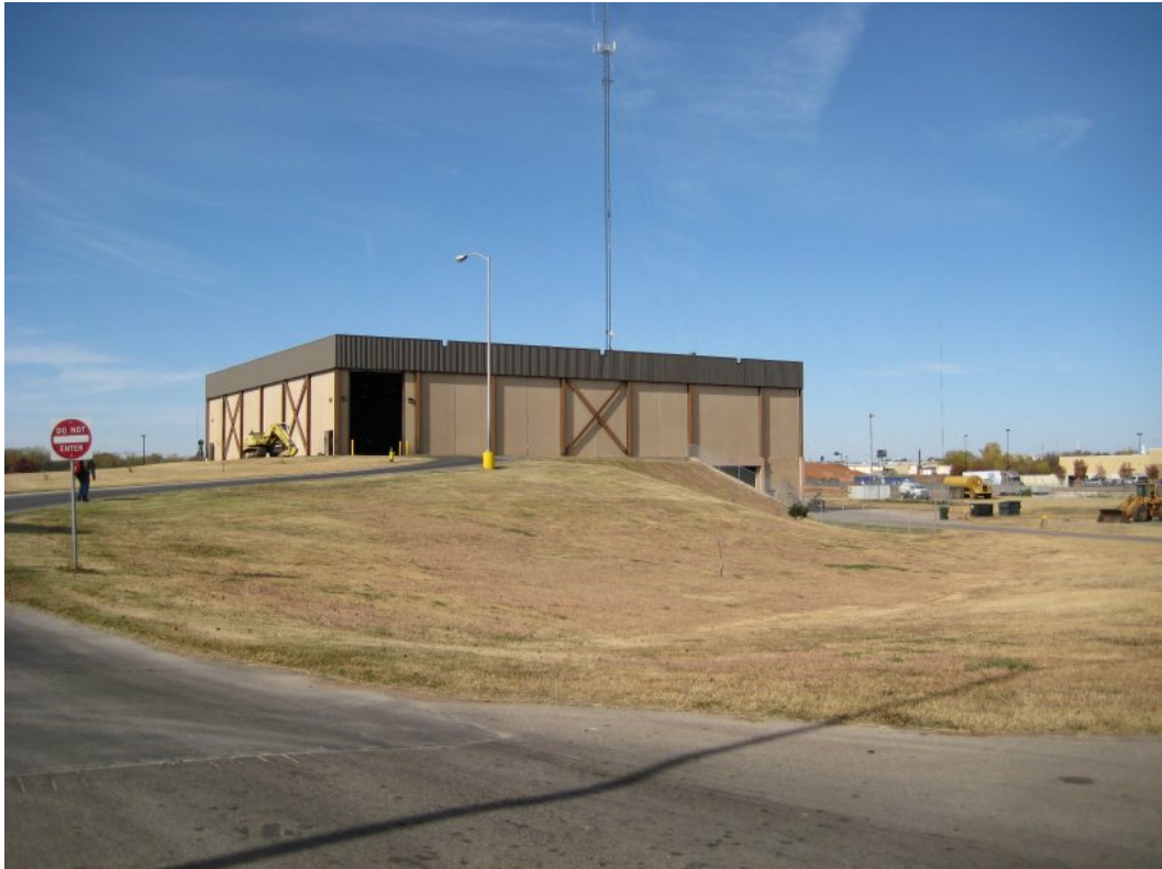
Figure 1-4. Transfer Station Building
