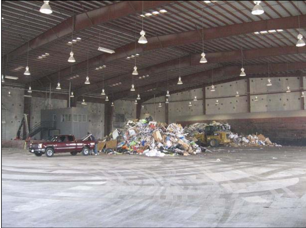
Figure 4-3. Transfer Station Tipping Floor
