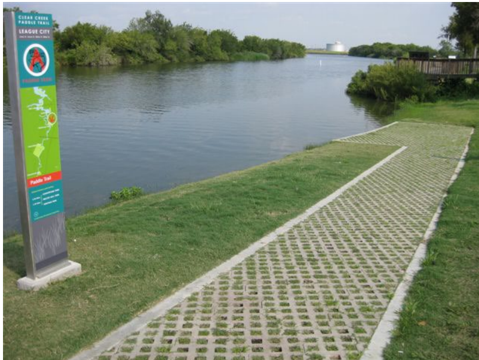
Figure 54 - WPP forms a pathway to a cleaner Clear Creek
