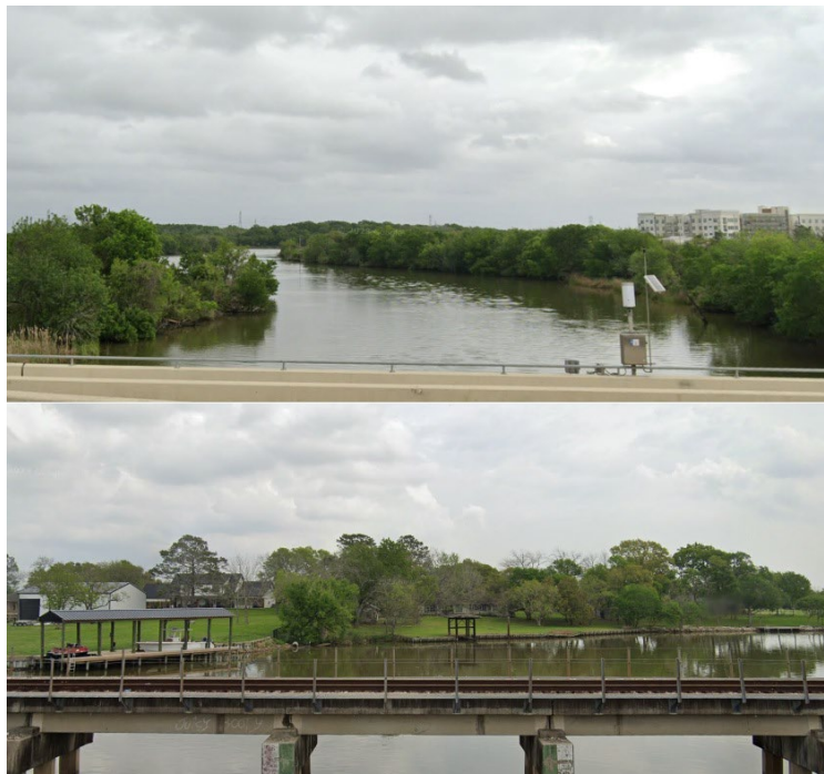
Figure 9 - Clear Creek at I-45 (top) and SH3 (bottom)
