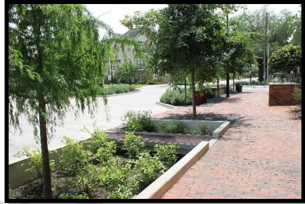
Figure 10. Curb cuts and biofiltration trenches along Bagby Street, Houston, TX 11
