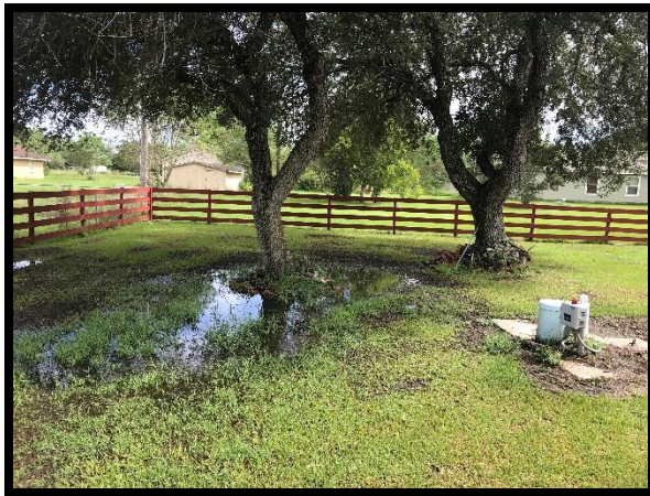
Figure 4. Failing onsite sewage facility
