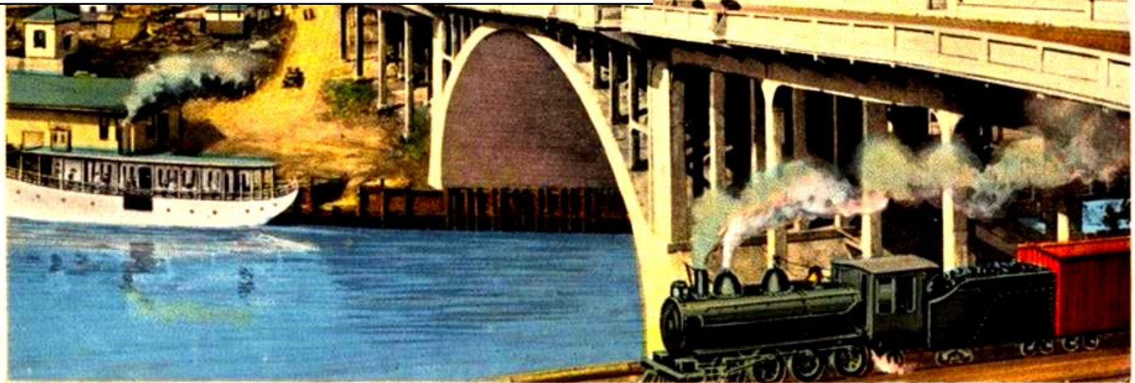
MAIN STREET VIADUCT AND SHIP CHANNEL, HOUSTON, TEXAS.
