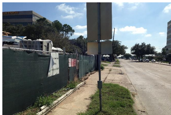
Image 14: Sidewalk along N. Dairy Ashford Road Facing South
