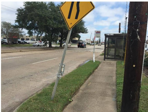
Image 15: Sidewalk along Memorial Drive Facing East
