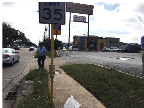
Image 22: Sidewalk along N. Dairy Ashford Road Facing South
