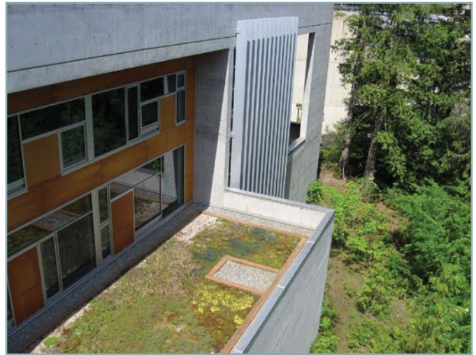
Figure 1: A green roof at Evergreen College was built to offset the addition of new impervious surfaces from new parking spaces.
