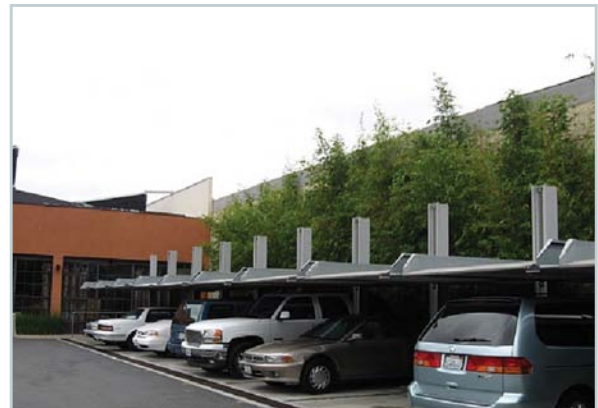
Figure 5: All developers in Emeryville, California, must comply with the City's "Stormwater Guidelines for Green, Dense Redevelopment," which requires green infrastructure, such as this stacked parking lot, throughout a project's planning and operation.
