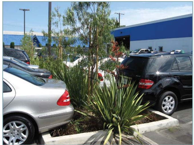
Figure 1: This commercial site includes parking lot swales to bioinfiltrate impervious surface runoff.
