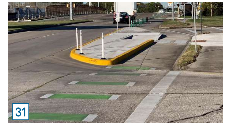
FIGURE 4.31 INTERSECTION CONFLICT MARKINGS, HOUSTON, TX
