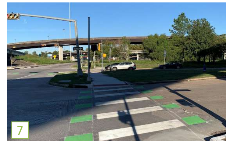
FIGURE 4.7 SHARED CROSSING PAVEMENT MARKING, HOUSTON, TX
