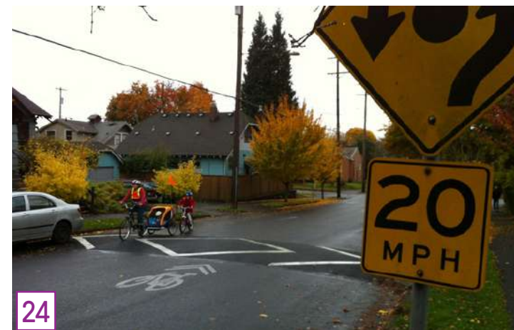
24 FIGURE 4.24 SPEED HUMPS, PORTLAND, OR
