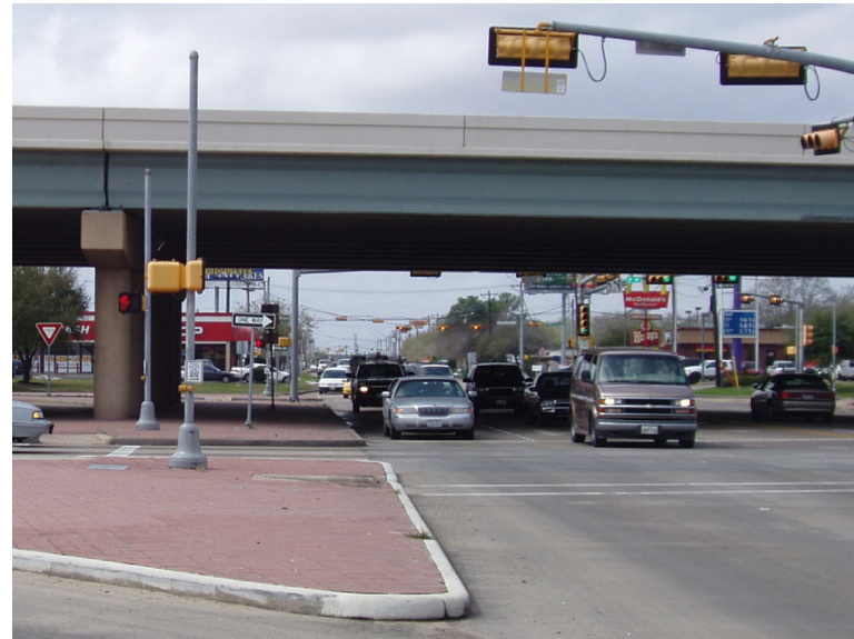
Exhibit 6.3-26: South Side of FM 518 Looking West through IH-45 (showing building close to ROW)
