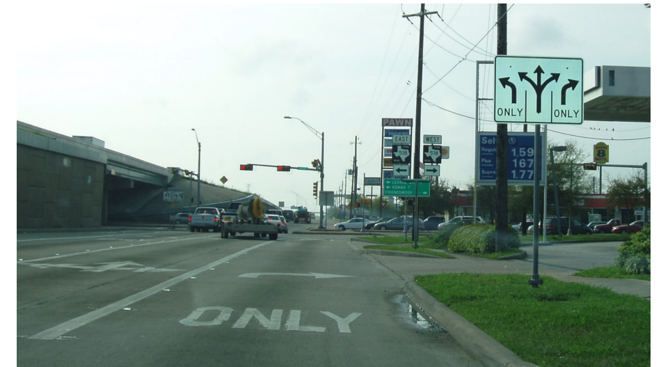
Exhibit 6.3-25: Existing Southbound Approach on IH-45 at FM 518
