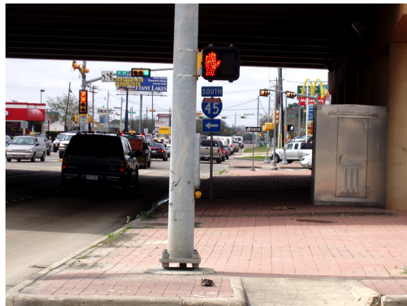
Exhibit 6.3-27: North Side of FM 518 at IH-45 (showing the existing TxDOT communications cabinet)
