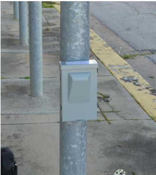
Installed counter without a lock.
