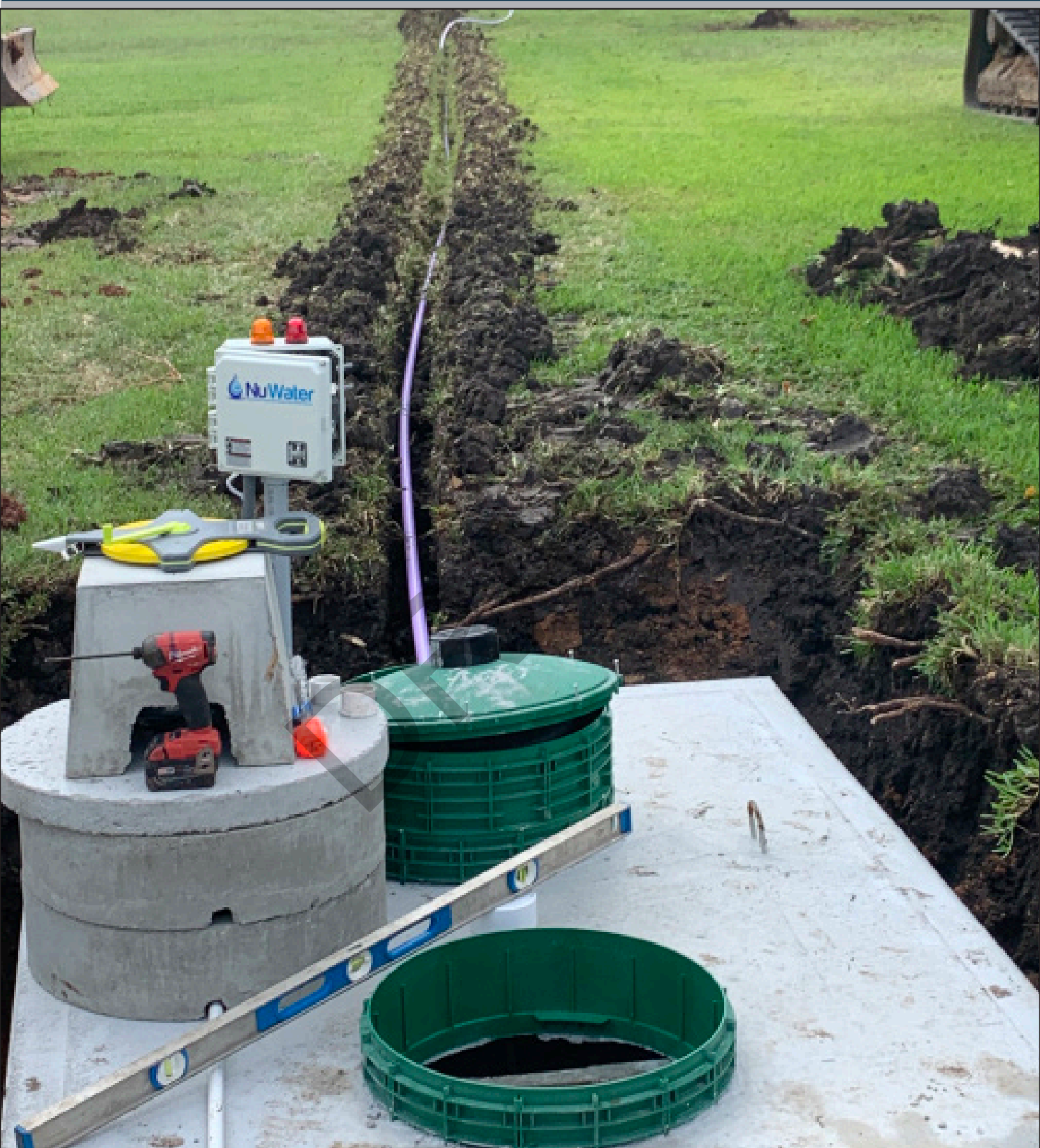
PHOTO: Installation of a new aerobic treatment unit
