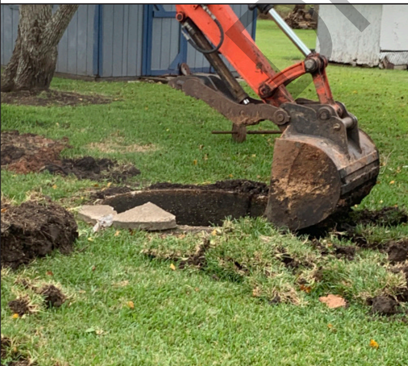
PHOTO: Decommissioning of a conventional septic system
