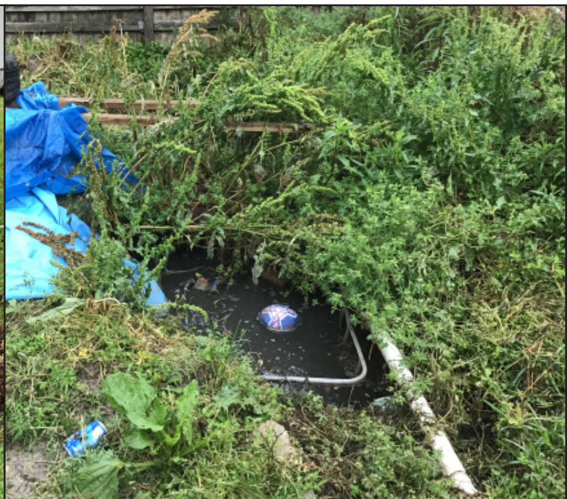
PHOTO: Surfacing sewage from a failed on-site sewage system
