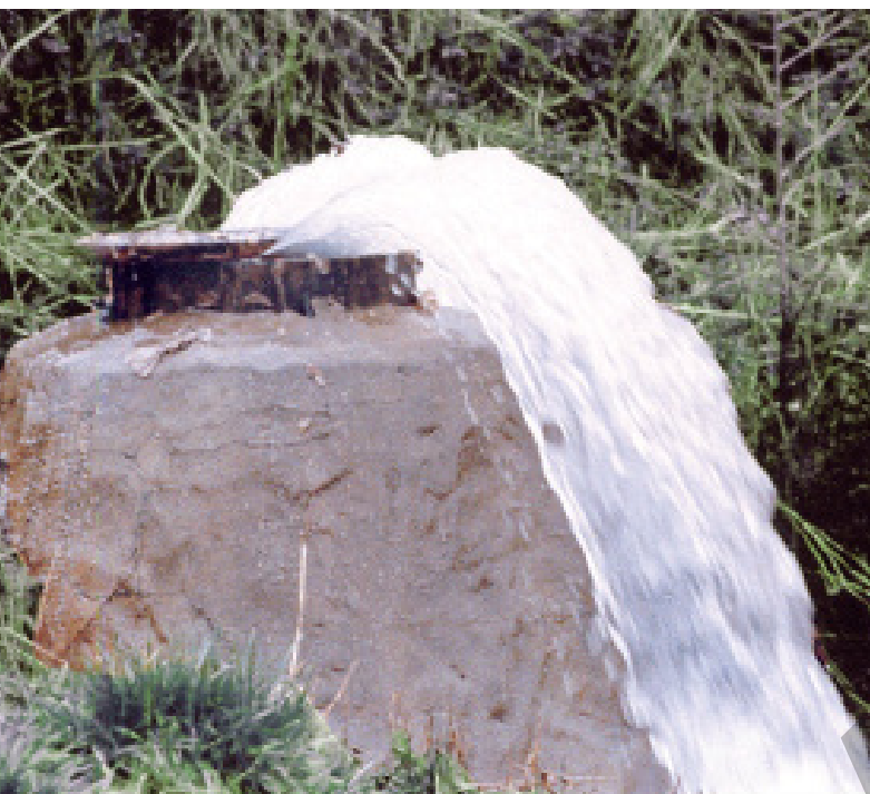
PHOTO: Sanitary Sewer Overflow
