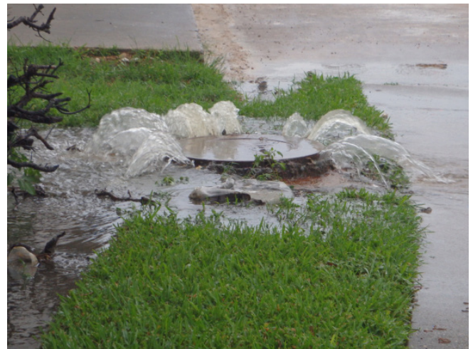
PHOTO: Sanitary Sewer Overflow
