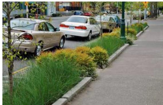
**Figure 5.21:** Bioswale and sidewalk
