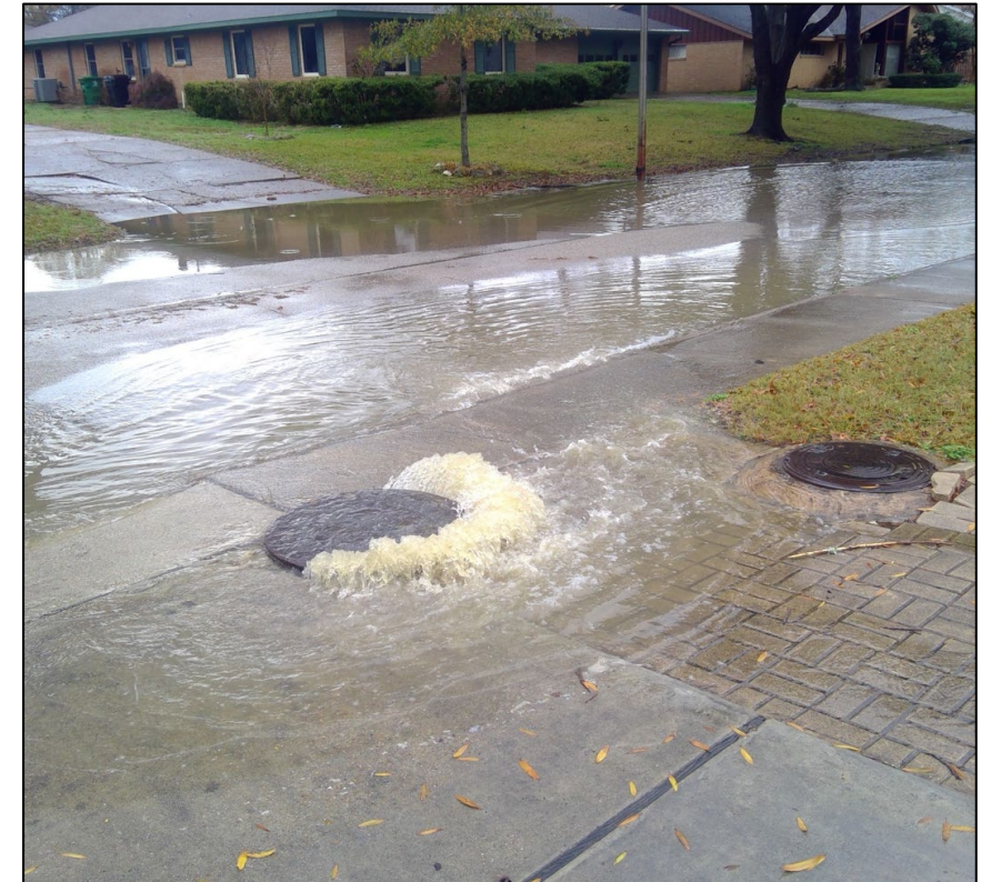
Sanitary Sewer Overflow ( SSO )
