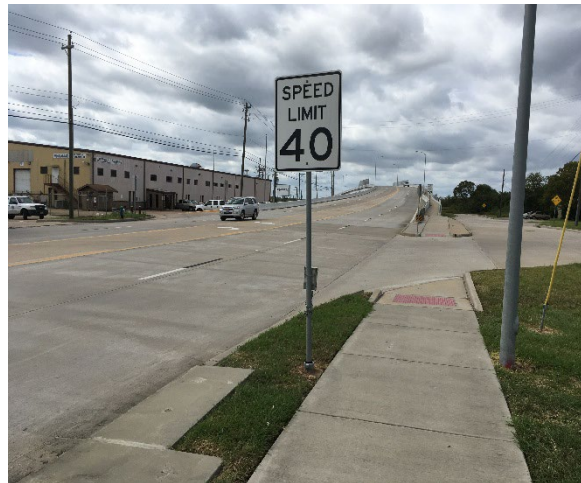
Sidewalk on Magnolia Road WB facing west
