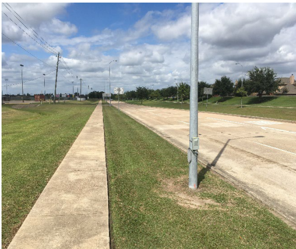
Sidewalk on Pearland Pkwy SB facing north
