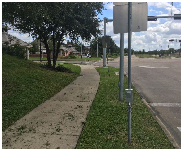
Sidewalk on Pearland Pkwy NB facing south
