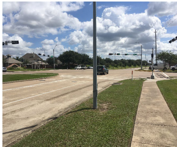
Sidewalk on Pearland Pkwy SB facing south
