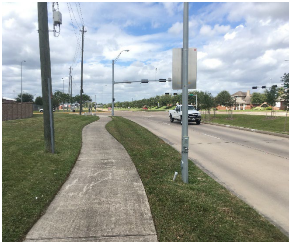
Sidewalk on Pearland Pkwy SB facing north
