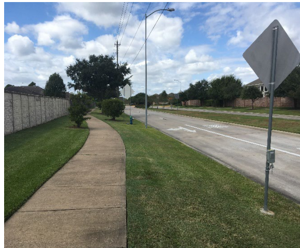
Sidewalk on Magnolia Road EB facing west
