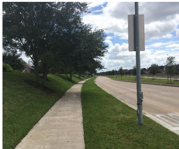
Sidewalk on Pearland Pkwy NB facing south
