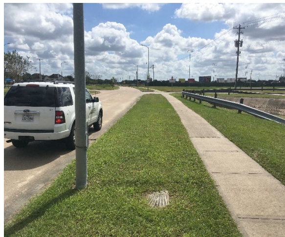
Sidewalk on Pearland Pkwy SB facing south
