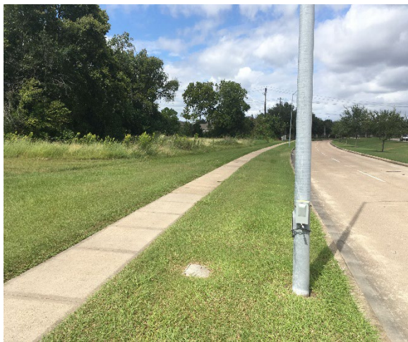
Sidewalk on Pearland Pkwy SB facing north
