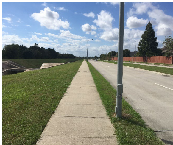
Sidewalk on Magnolia Road EB facing west
