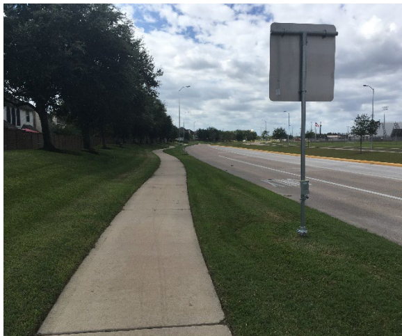
Sidewalk on Oiler Drive EB facing west
