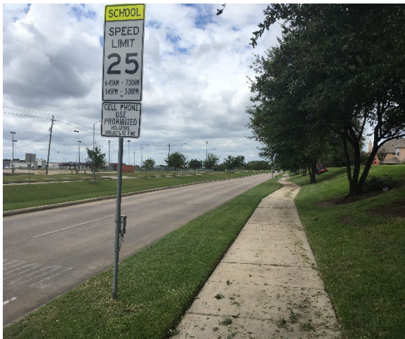
Sidewalk on Pearland Pkwy NB facing north
