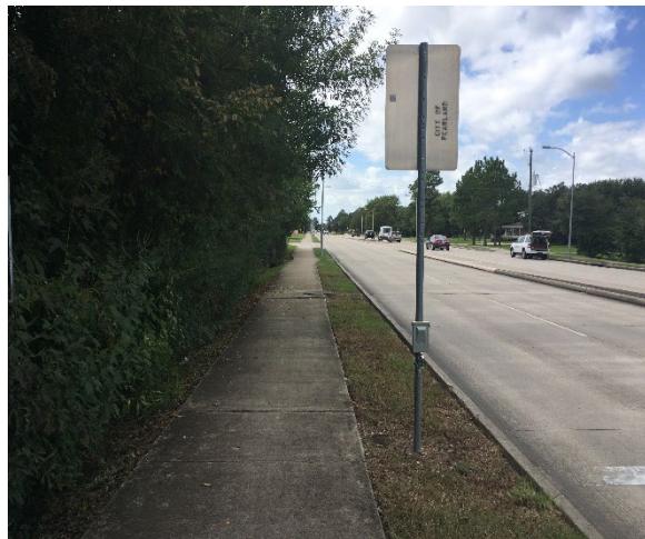
Sidewalk on Magnolia Road EB facing west
