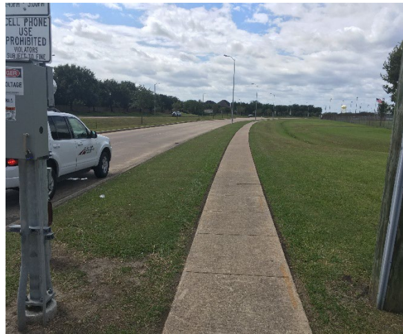
Sidewalk on Oiler Drive WB facing west
