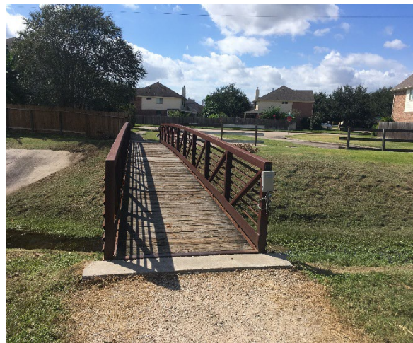
West Oaks Trail Bridge facing west
