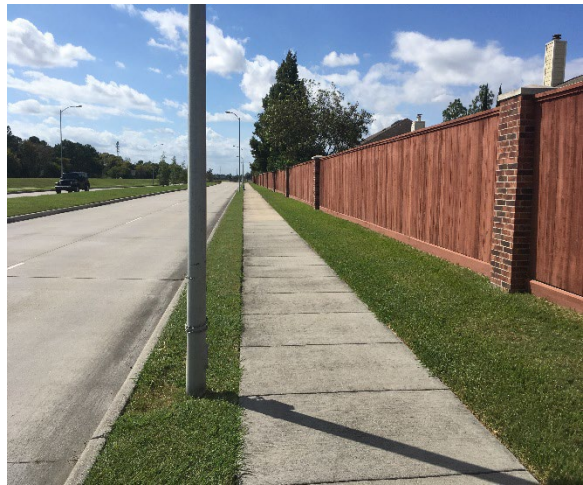
Sidewalk on Magnolia Road WB facing west
