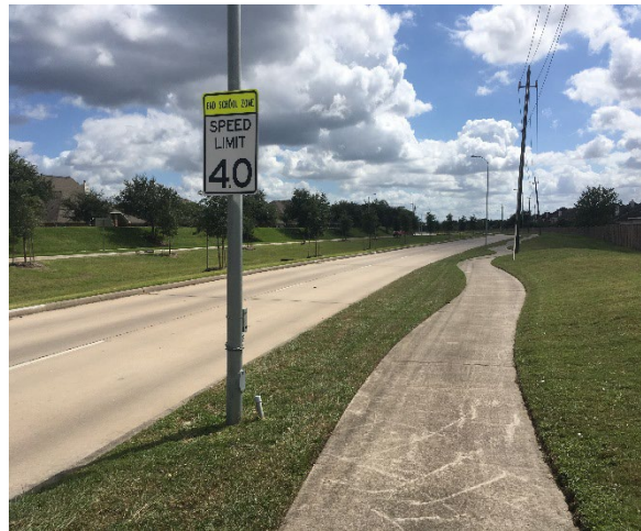
Sidewalk on Pearland Pkwy SB facing south
