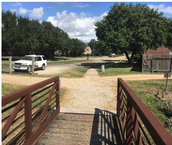
West Oaks Trail Bridge facing east
