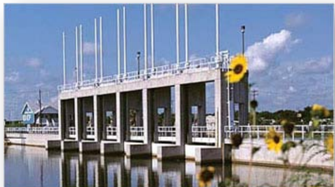
Figure 23. Clear Creek second outlet channel floodgates
