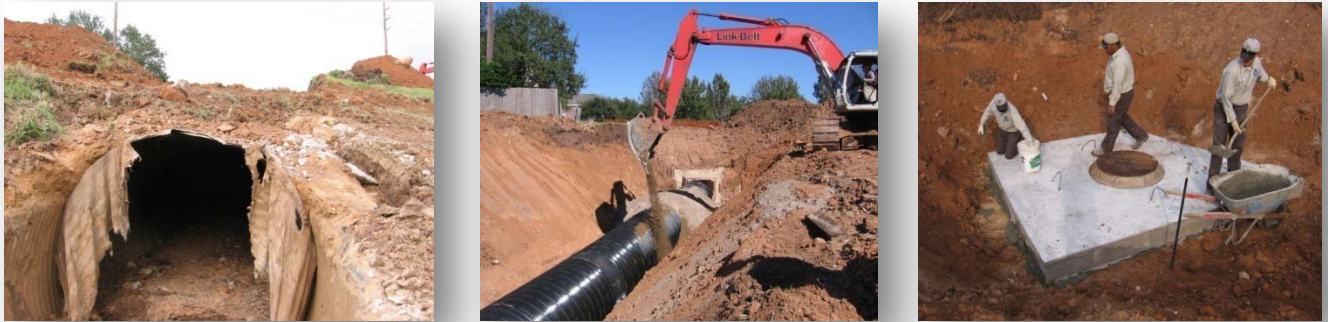
Figure 9. Collapsed storm sewer outfall and subsequent repairs.
