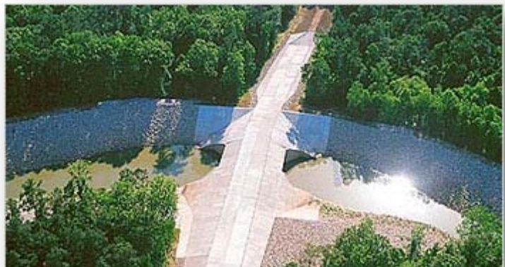
Figure 14. Detention basin control structure in the Greens Bayou watershed
