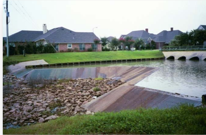
Figure 18. Dam, in Missouri City, designed to maintain the water level upstream and mitigate flooding downstream
