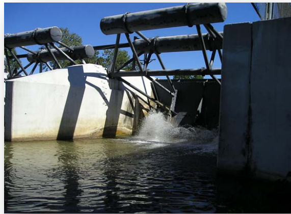
Figure 23. AMIL Gates in the City of Sugar Land divert flood waters and protect the city
