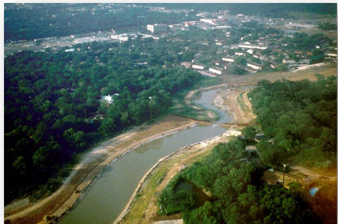
Figure 34. Corps project at Sims Bayou
