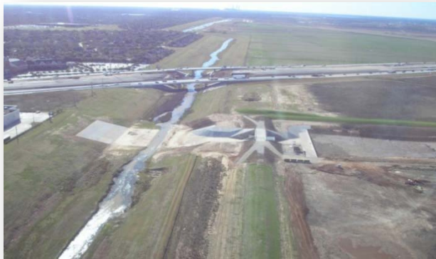
Figure 22. Levee and stormwater pump station in the City of Sugar Land
