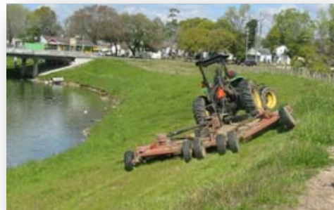
Figure 8. The slope is mowed to maintain function at an optimal level.
