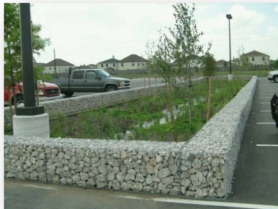
Figure 30. This bio-swale is located in the parking lot of the Gene Green Park off Beltway 8 in northeast Harris County.
