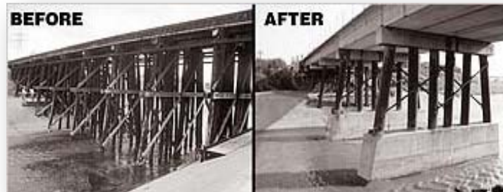
Figure 10. Railroad bridge modifications reduce flow restrictions and as a result reduce the effect on future flood waters.
