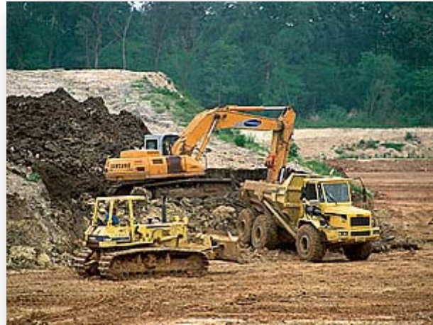
Figure 26. Fill is removed from the floodplain to compensate for fill added
