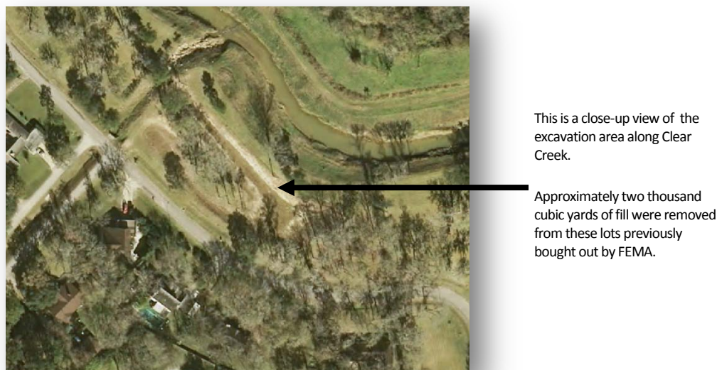
Figure 16. Close-up of area excavated
