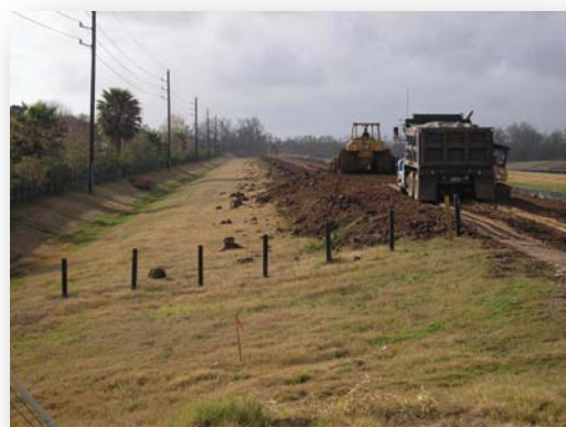
Figure 21. Levee reconstruction work
