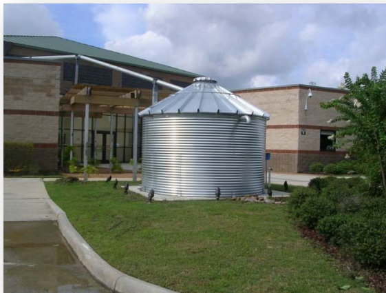
Figure 29. This cistern catches rainwater from the rooftop of the City of Houston Northeast Water Production Plant and is then used to water the landscaping on site.
