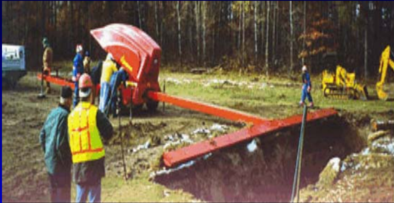
T-400 Trench Burner and Pit Construction (Minnesota)
