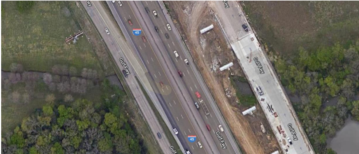
Figure 29 - Unnamed Tributary Passing Beneath I-45 at Station 18591
