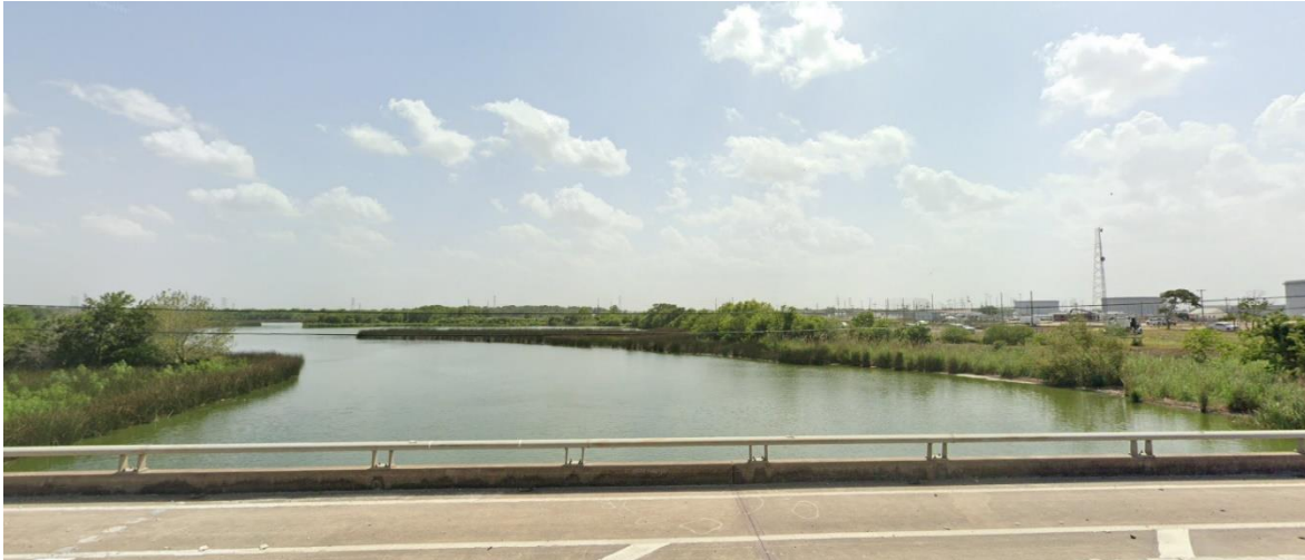
Figure 32 - Clear Creek Tidal at State Highway 3
