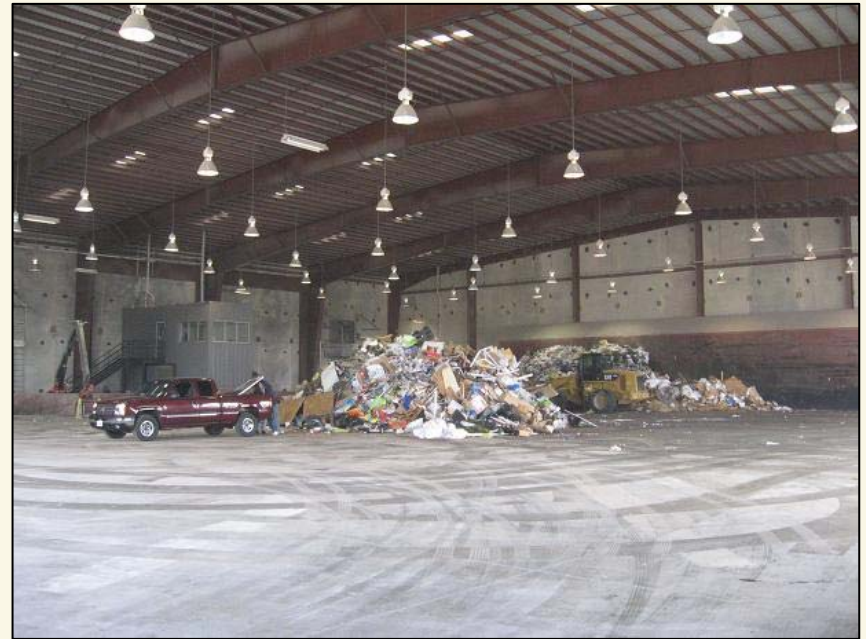
Transfer Station Tipping Floor
