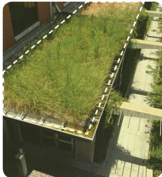
Green Roof, Houston Permitting Center
