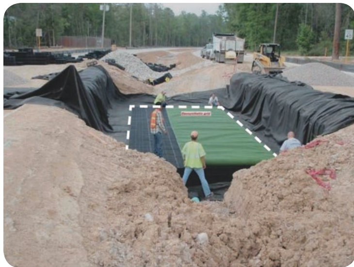
Underground storage tank, Birnamwood Drive
