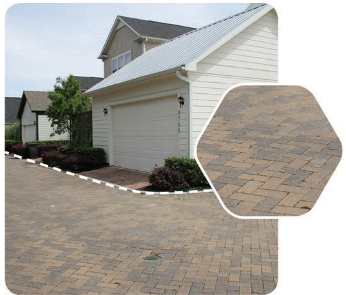
Permeable Pavement, Kempwood Manor
