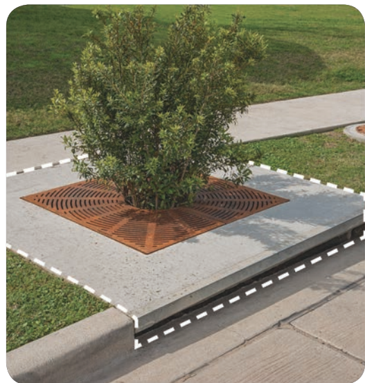
Stormwater Planter Box, Darling Street
