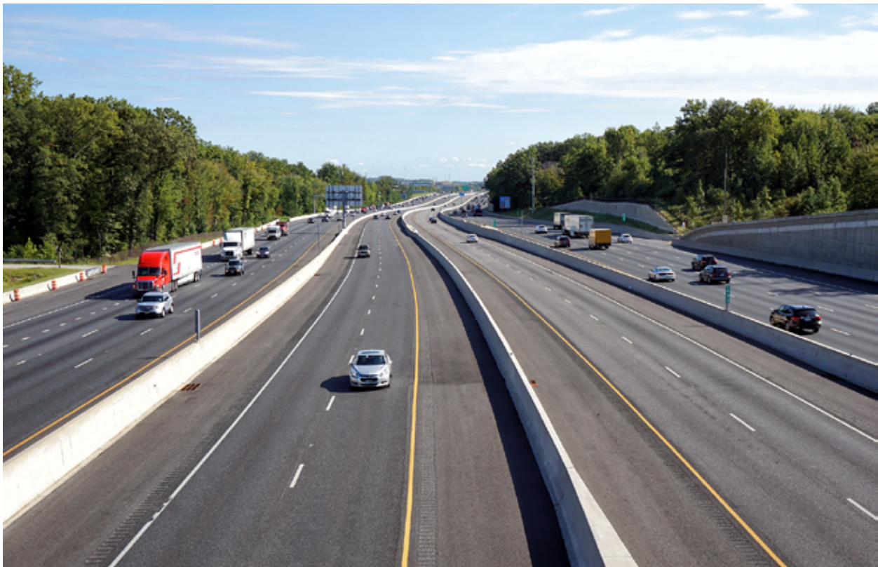
The Interstate 95 Express Toll Lanes in Baltimore, opened in 2014, feature high design standards with concrete barrier separation and full shoulders. Photo: AsphaltPlanet.ca.
