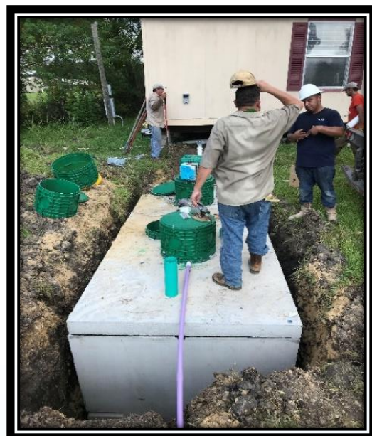
Figure 4. Onsite sewage facility replacement
