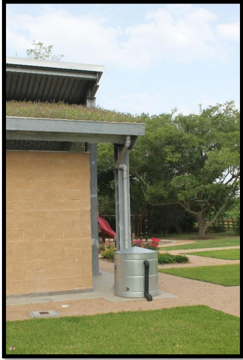
Figure 11. Green roof and rain barrel, Ghirardi Watersmart Park, League City, TX 12
