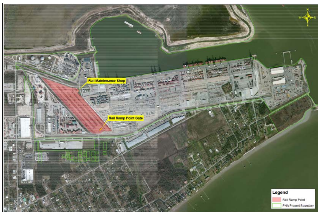
Figure 4-8. Rail Ramp at Barbour's Cut
