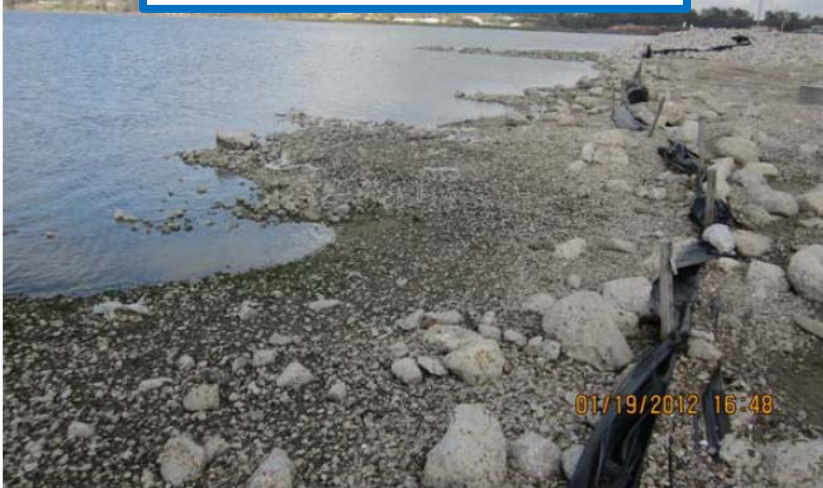
Photo: 48 Silt fencing along the northern shoreline of the Western Cell (view northeast)
