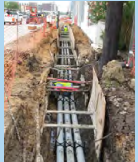
Improved Kirby Drive streetscape, courtesy Gunda Corporation Underground utility ducts, construction phase
