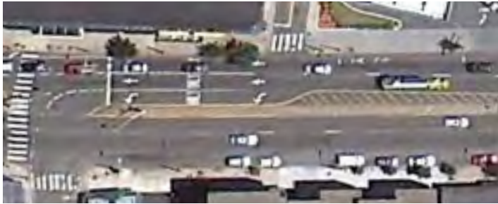
Traffic flow is directed with painted lines rather than a built median, allowing for a testing period in lane alignment, which may be built or adjusted accordingly.
