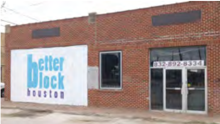
one of the vacant storefronts that the project activated
