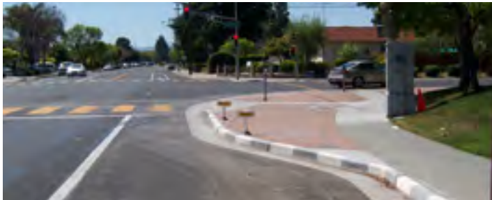
Sidewalk extension (bulb-out) defines the parking lane and improves the pedestrian realm.
