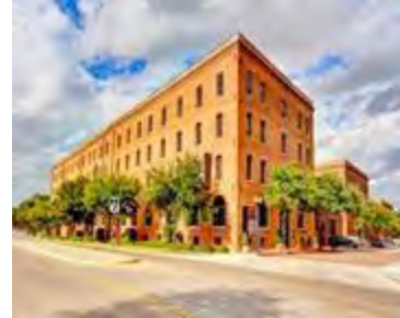
3 East End Lofts
