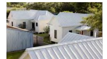
16 The Plant House
