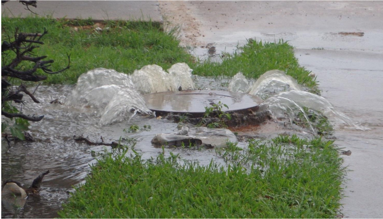
Figure 29 - SSO in progress
