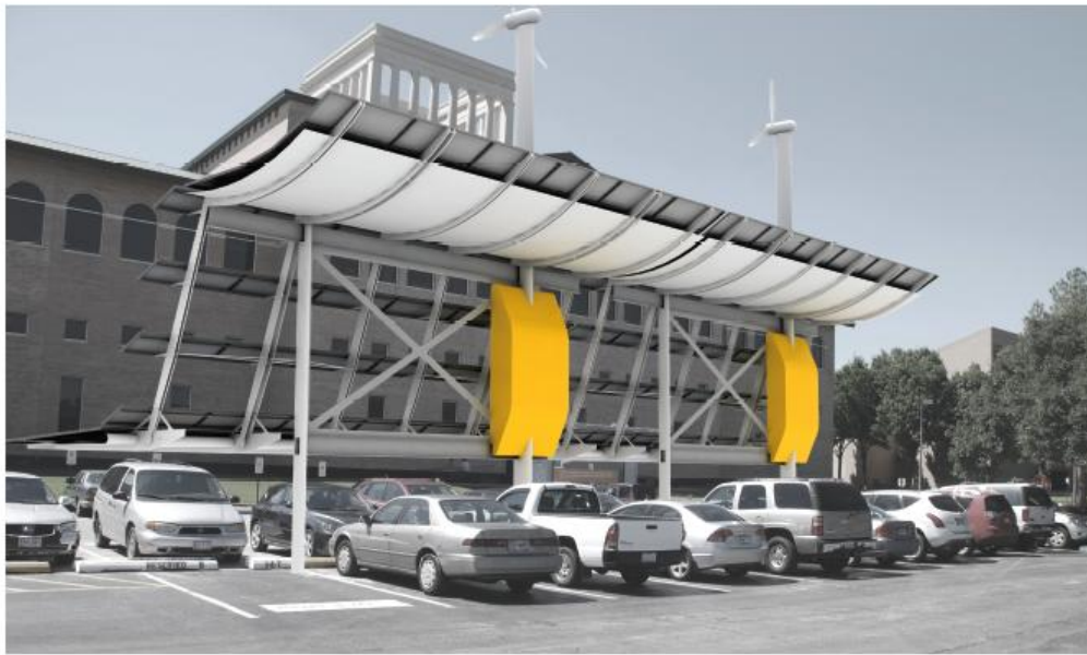
VIEW OF ELEVATED CISTERNS AND WATER CATCHMENT PANS
