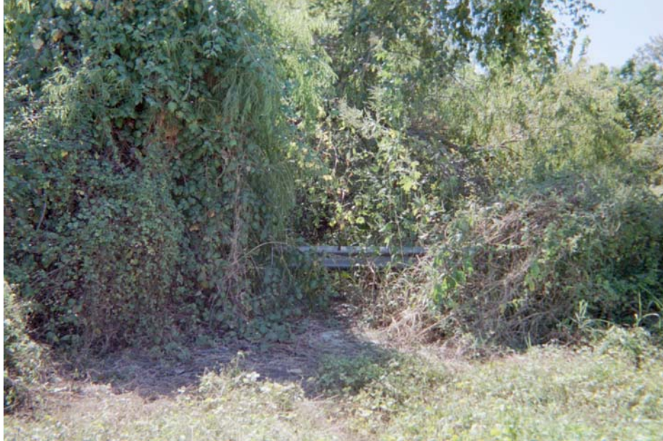
Photo 10-1 Site 16649, picture taken from bridge facing northeast. Heavy vegetation and fences blocked access to stream bank at Clinton St.
