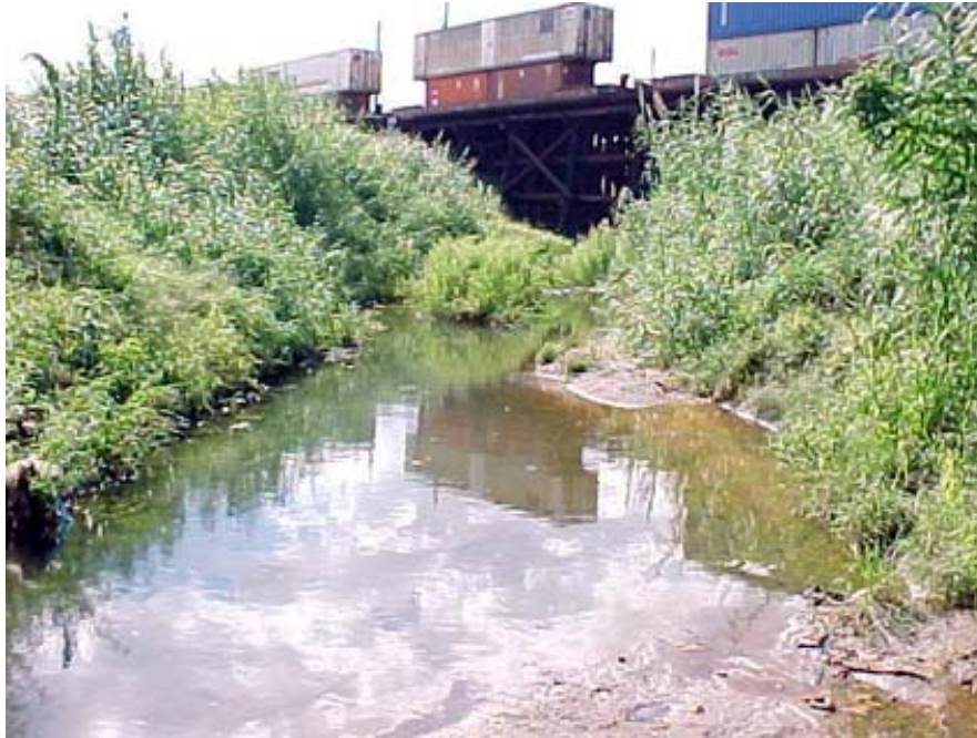
Photo 8-3 Site 16651, picture taken from bank facing east.
