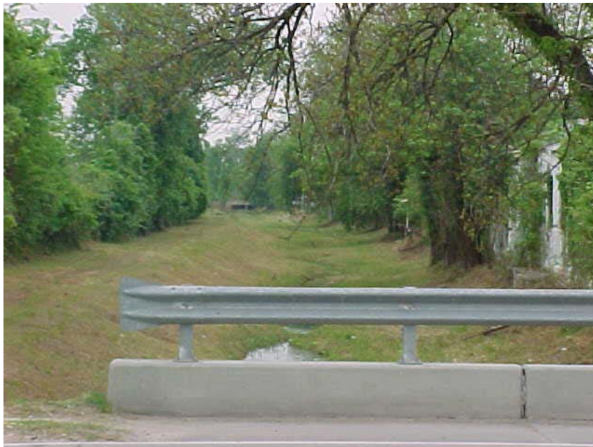
Photo 9-5 Site 15867, North fork of Hunting Bayou east of US-59, looking west of Jensen Dr. upstream of the confluence with south fork. The far end of channel passes into a culvert and under railroad tracks.
