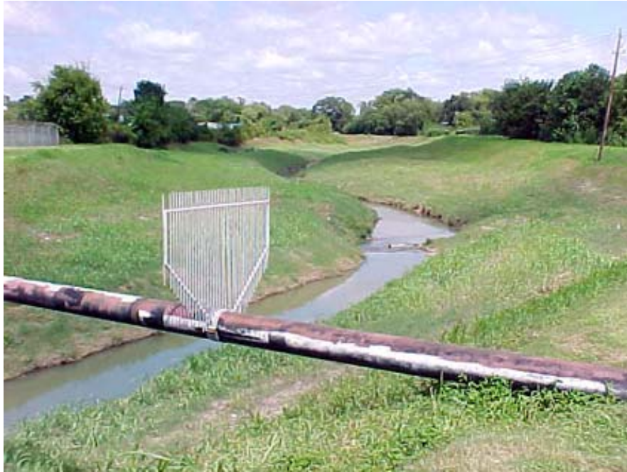
Photo 9-1 Site 11129, picture taken from bridge facing northeast.
