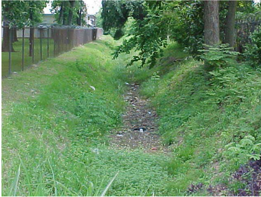
Photo 10-3 First open channel found on 1007O south of IH 10 looking South from Sonora St. to channel. Industrial complex on left, residences on right. Finnigan Park is located beyond houses, approx. 200 feet to the right of this photo.
