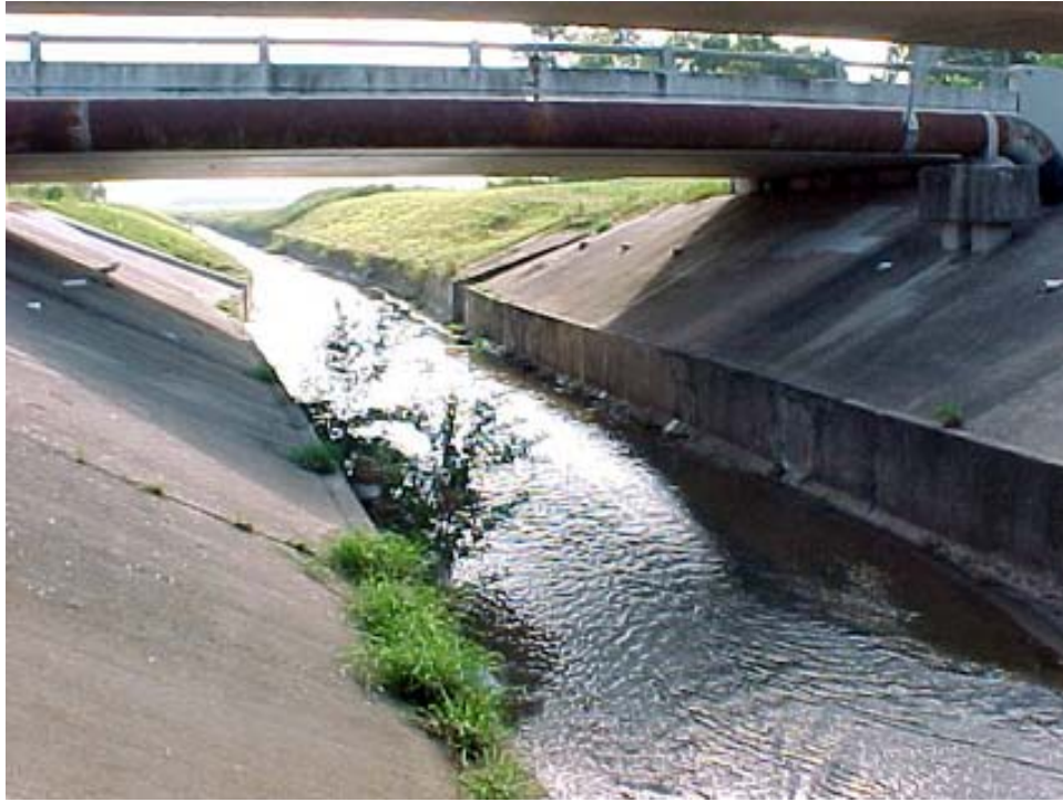
Photo 4-3 Channel C-147 tributary to Sims Bayou Site 15875. picture taken from bank facing east.
