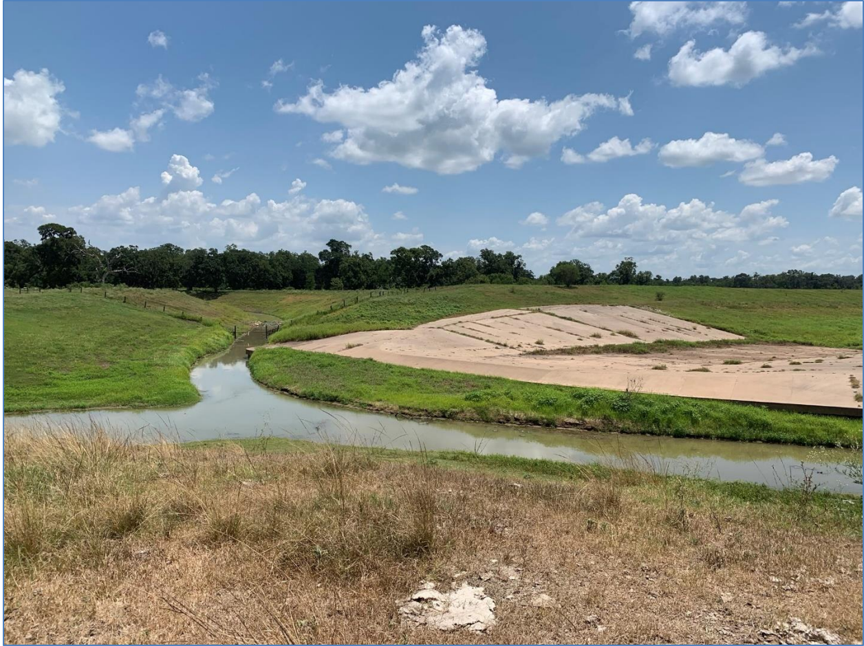
Figure 8 - Drain Bypass Structure at the Confluence of Rabbs Bayou and Big Creek
