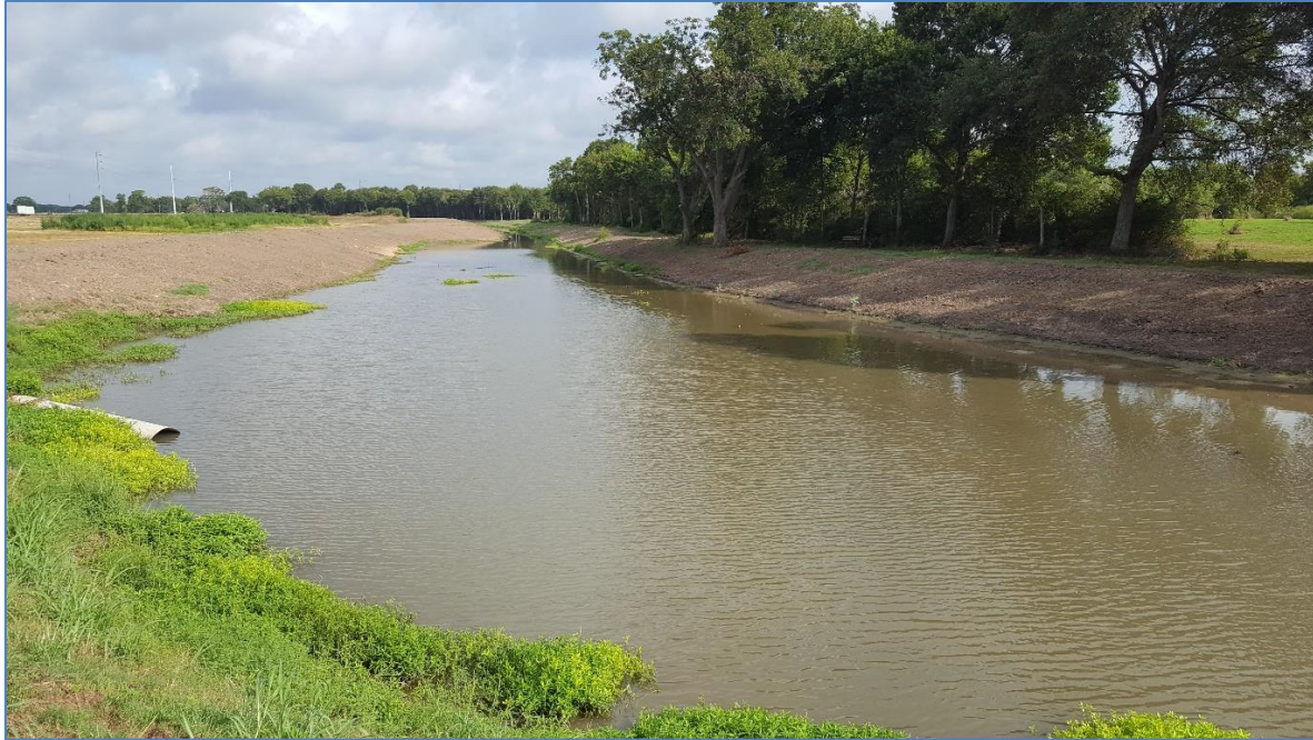
Figure 13 - Stormwater Management Structure near Seabourne Creek Park
