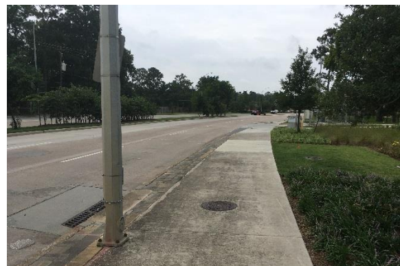
Image 6: Sidewalk along Eldridge Parkway Southbound at Energy Center IV Facing South
