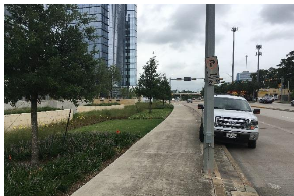
Image 5: Sidewalk along Eldridge Parkway Southbound at Energy Center IV Facing North
