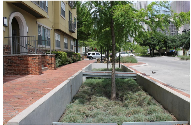
Figure 7. Bioswales with curb inlets along Bagby Street, Houston
