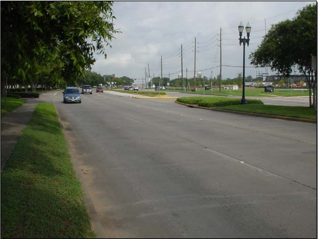
Figure 5-1: Existing Sugar Land Photo
