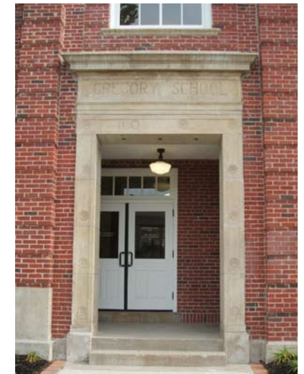
Welcoming entry points on both the north and south facades make the Library a welcoming and accessible facility.
