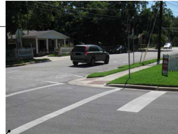
Basic painted crosswalks at ADA street crossings.
