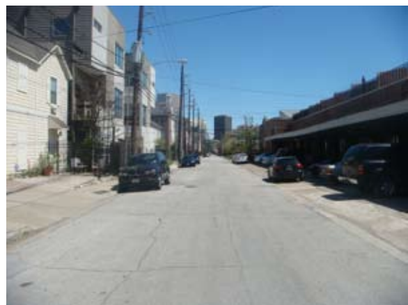
Diverse street conditions along West Webster Street
