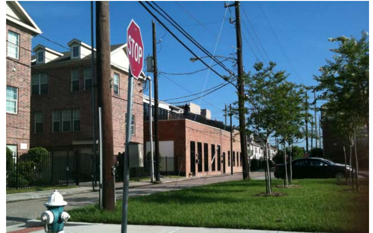
Some new construction includes trees (understory or ornamental) that provide meaningful shade and are “good neighbors” for overhead utilities.
