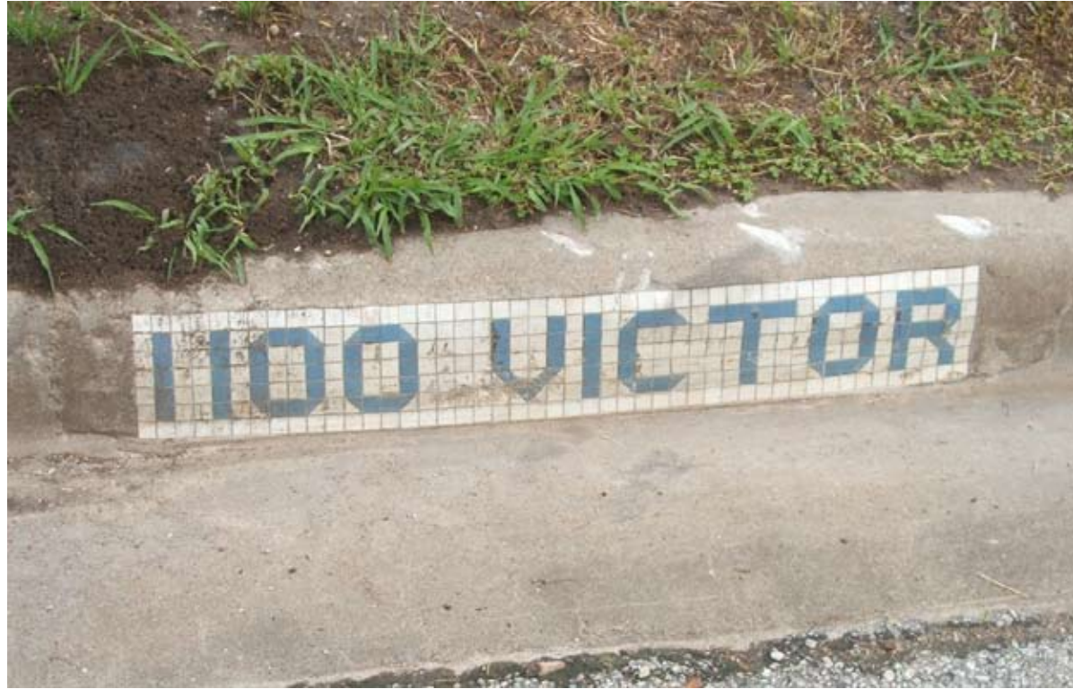
Tile street markers and block numbers provide a layer of wayfinding throughout the area. Many of these markers are in poor condition or missing.
