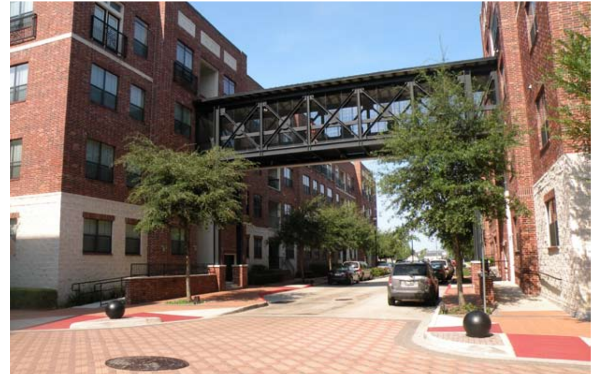
The Camden/Midtown redevelopment area has run all utilities underground, allowing room for trees to be planted and a general de-cluttering of the pedestrian environment.
