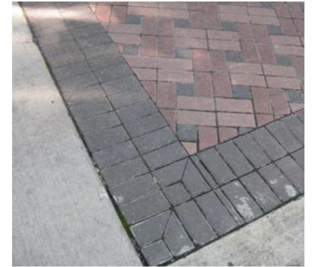
Pavers with a similar color palette to those used at Camden should be used for crosswalks as key nodes and entry points. Material selection should avoid mimicking historic brick and patterns.
