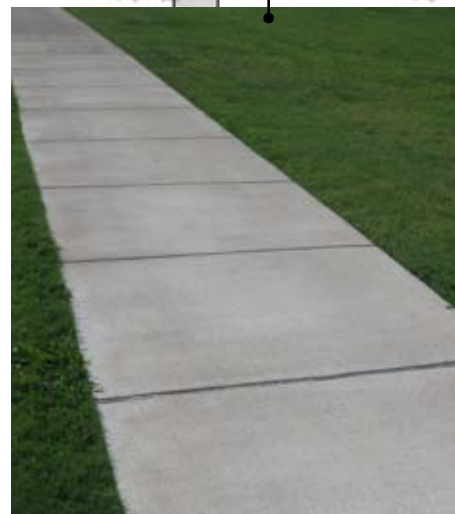
Basic concrete sidewalk and jointing.
