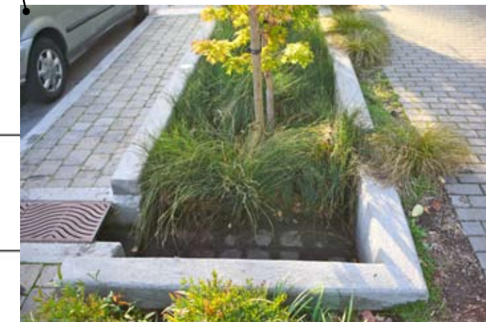
Stormwater filtration basin with raised curbs and plantings.
