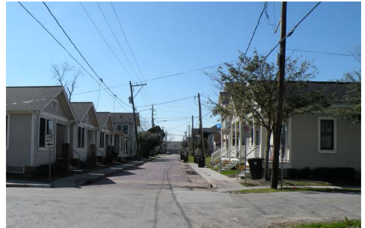
Most streets in the core of the study area are narrow, one-way roads due to historic land patterns and on-street parking demands.
