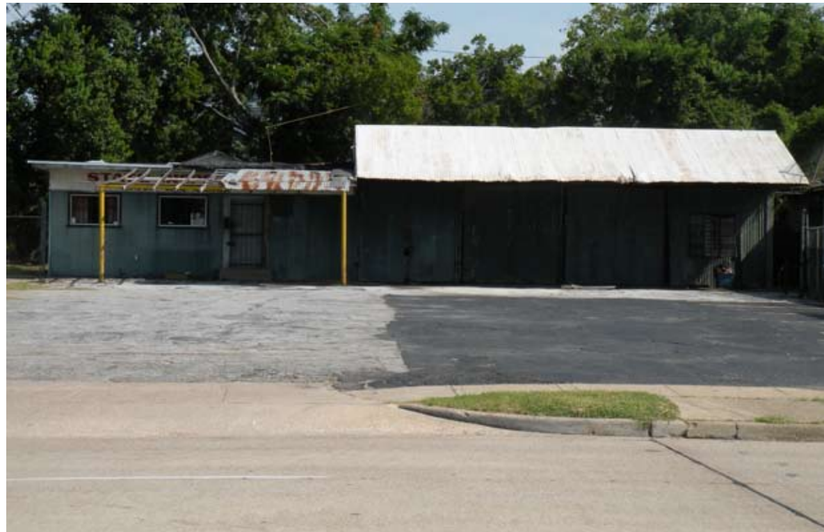
A few large parcels along West Gray are either vacant or undeveloped. These could provide major redevelopment opportunities (23).
