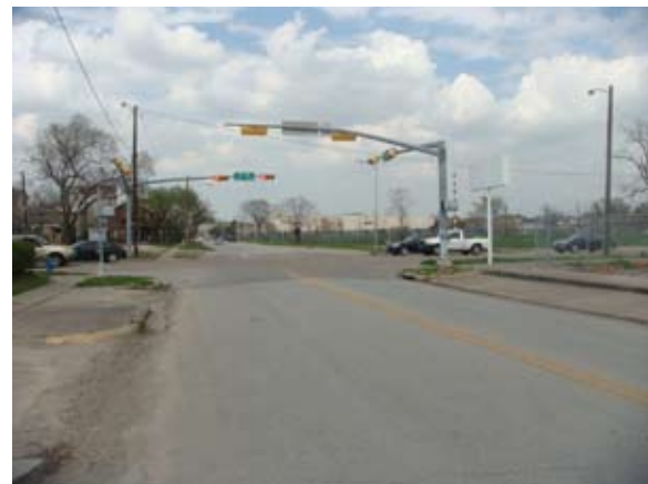
Taft Street bordered by the school site
