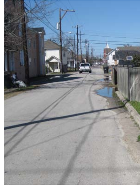
This photo depicts the conditions of a typical interior street within the study area. Narrow widths, utility poles, and various obstacles are constraints for the creation of pedestrian infrastructure.
