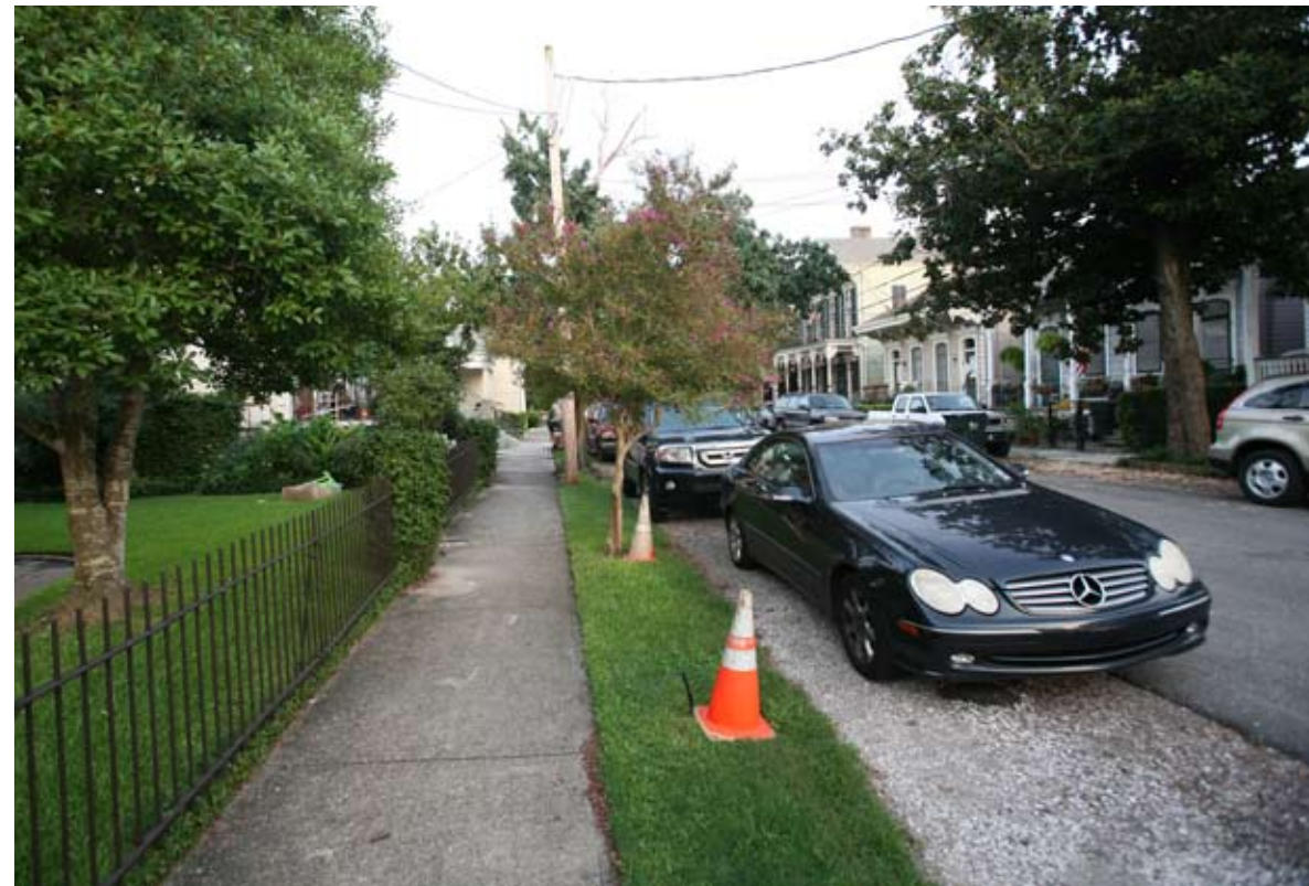
Narrow streets in New Orleans utilize an "overlapping systems" approach in many areas. This street includes a narrow roadway, expanded crushed shell shoulders for parking, ADA pedestrian path, and narrow planter/utility zone. Utilizing pervious materials reduces demand on drainage systems. (Photo: Algiers Point, New Orleans)
