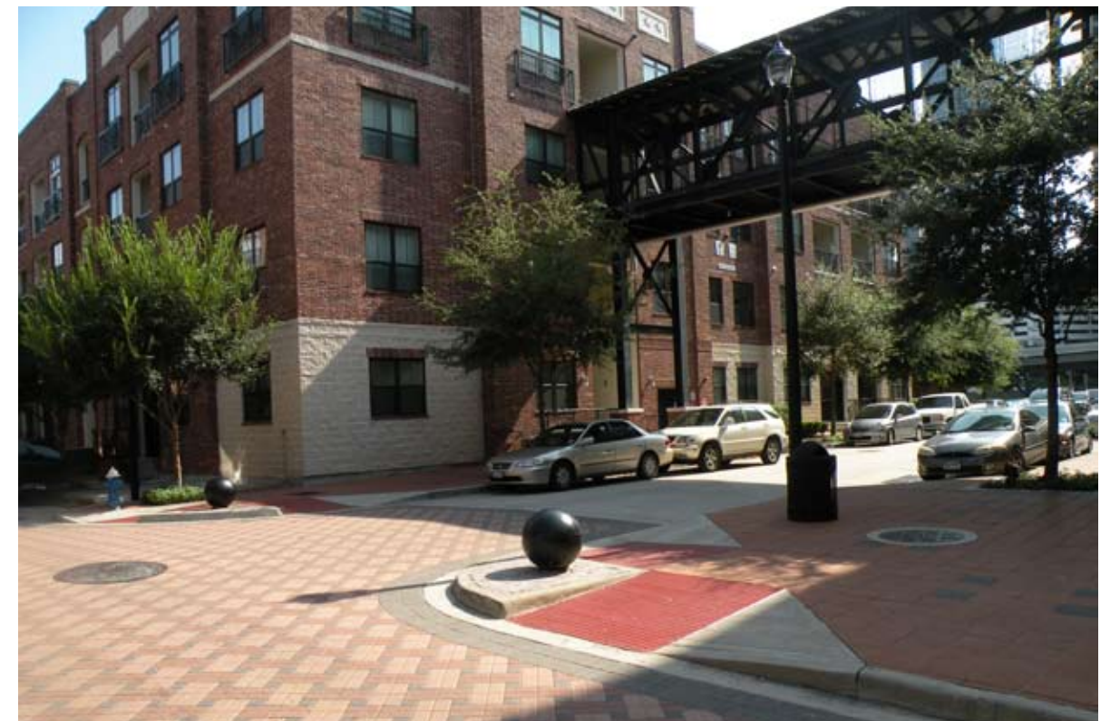
Camden represents a development pattern that is growing due to the success of Midtown. Although this type of development displaces endemic character, it also provides densities needed to support services and retail.
