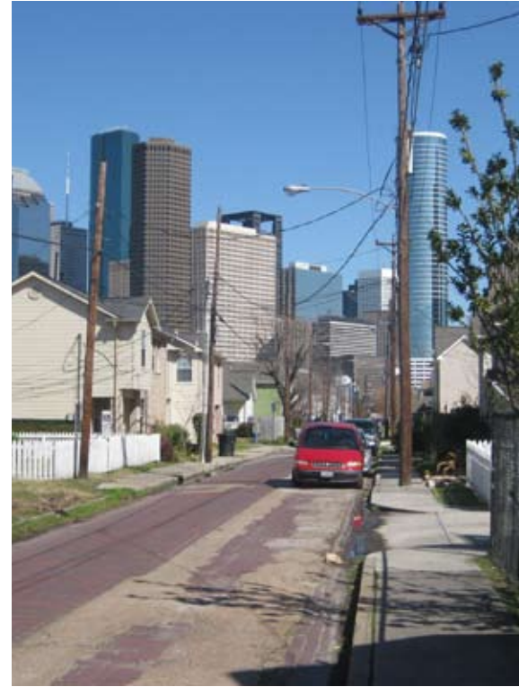
Overhead utility lines and narrow rights-of-way make adding trees and vegetation difficult.
