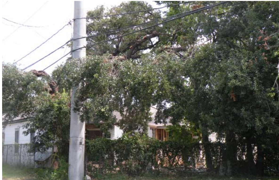
Conflicts between vegetation and overhead utilities often lead to heavy pruning and growth control by utility companies. This is not good for the general health of the plants, creation of shade, and operation costs of utility companies.
