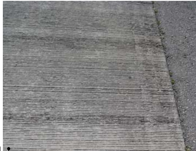
Wire or deep raked finish concrete next to a standard finish. Lines run perpendicular to traffic flow.
