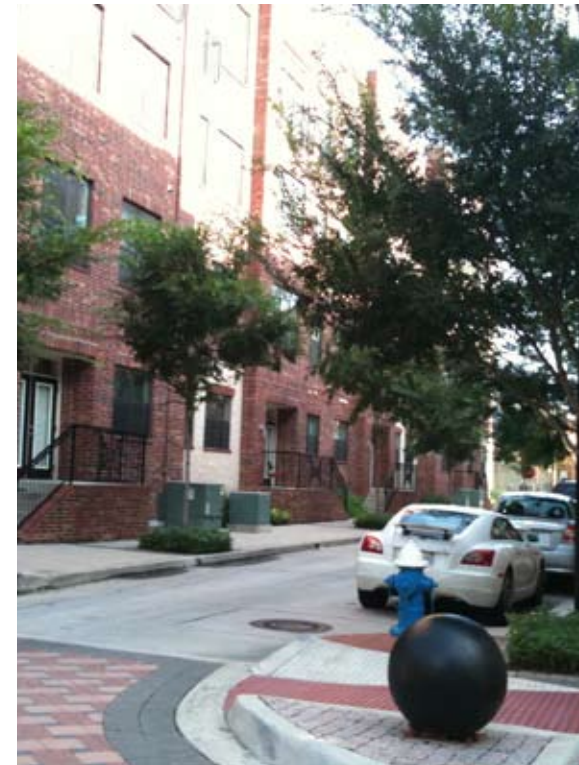
The Camden development buried power lines and created a usable pedestrian area.
