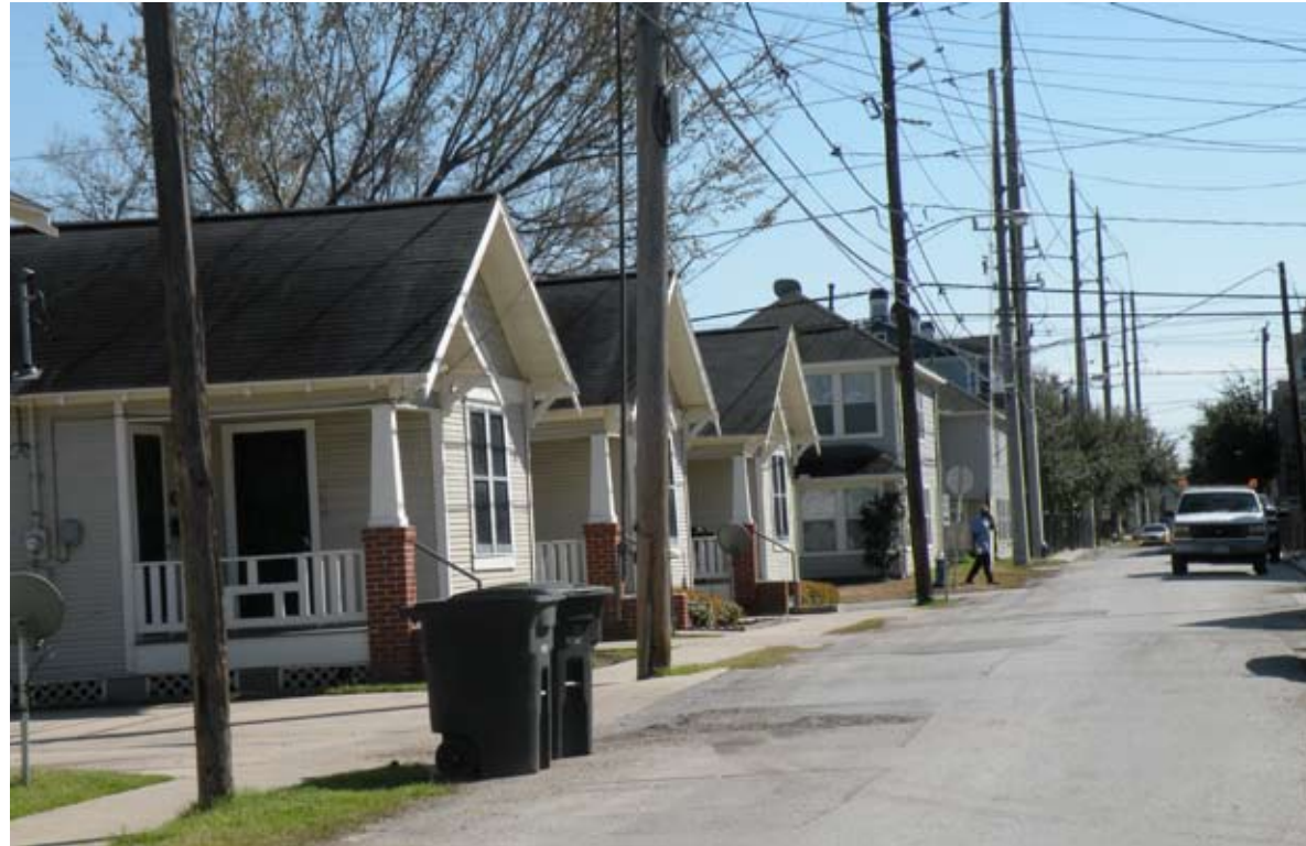
Overhead lines, poles, and accessories dominate the skyline in much of the study area resulting in a lack of vegetation along the street.
