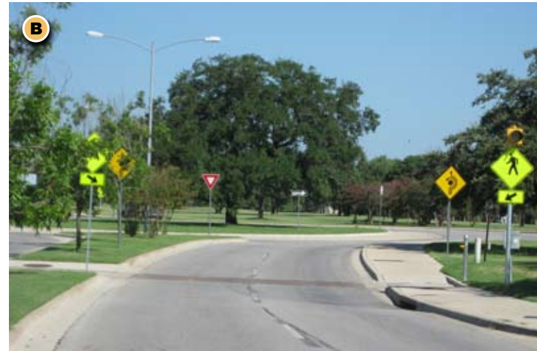
Pedestrian yield zones include flashing lights, pavement striping of some kind, and signage. Lights are only active when pedestrians are in the area.
