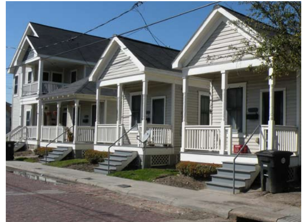
Encouraging on-street parking, better transit service, and development that is human-scaled will minimize parking demand in the neighborhood and create places that serve a diverse group of residents. (Photo: Ruthven Street)
