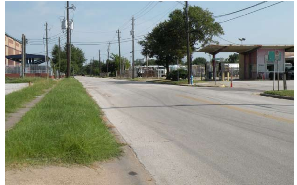
The Gillette Tract is the largest parcel of land owned by the City of Houston in the area. A redevelopment strategy for this site will be included in the overall approach for this project. Former City property adjacent to the tract is now owned by a private development team (9).
