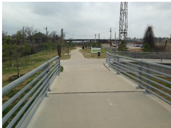
Image 14: Bridge over White Oak Bayou Facing West
