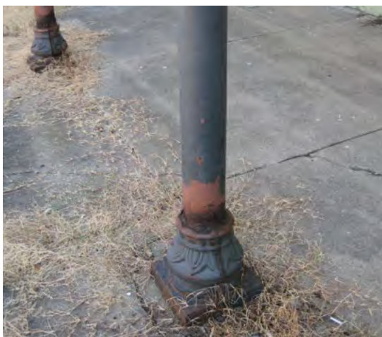
[7] (a) After the damaged portions of the base were repaired, (b) the cast-iron columns were cleaned and repainted to protect the metal from rusting.
