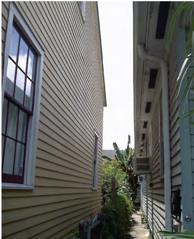
[9] Smooth-surfaced cementitious siding (left) may be used to replace deteriorated wood siding only on secondary elevations that have minimal visibility.
