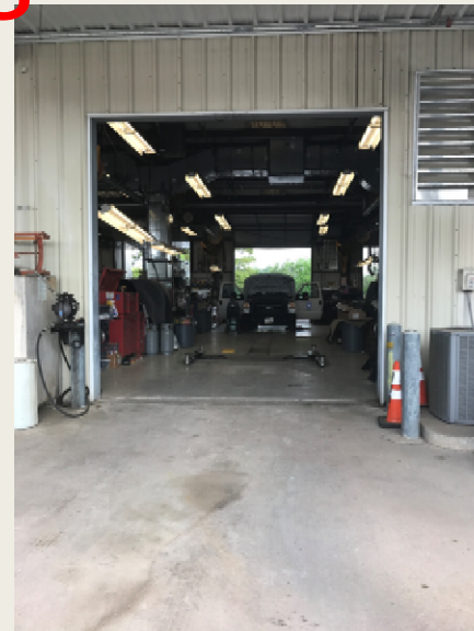
Cleaned area and installed oil water separator drainage system.
