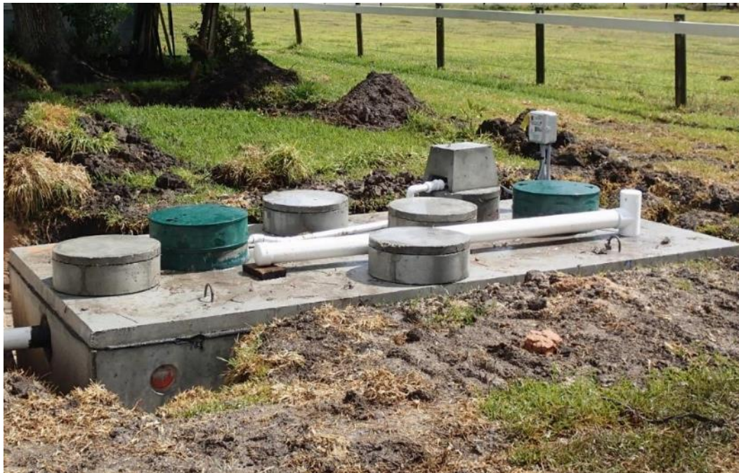
Figure 59 - OSSF being installed
