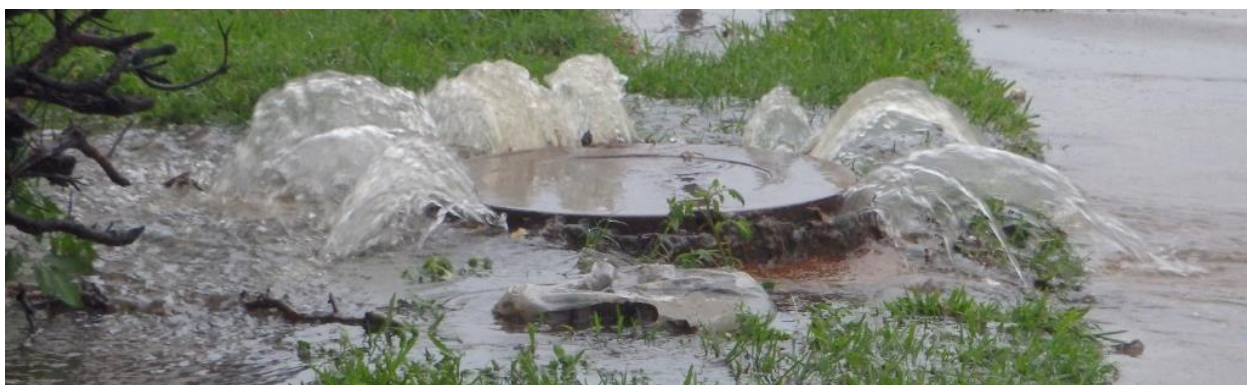
Figure 26 - SSO in progress
