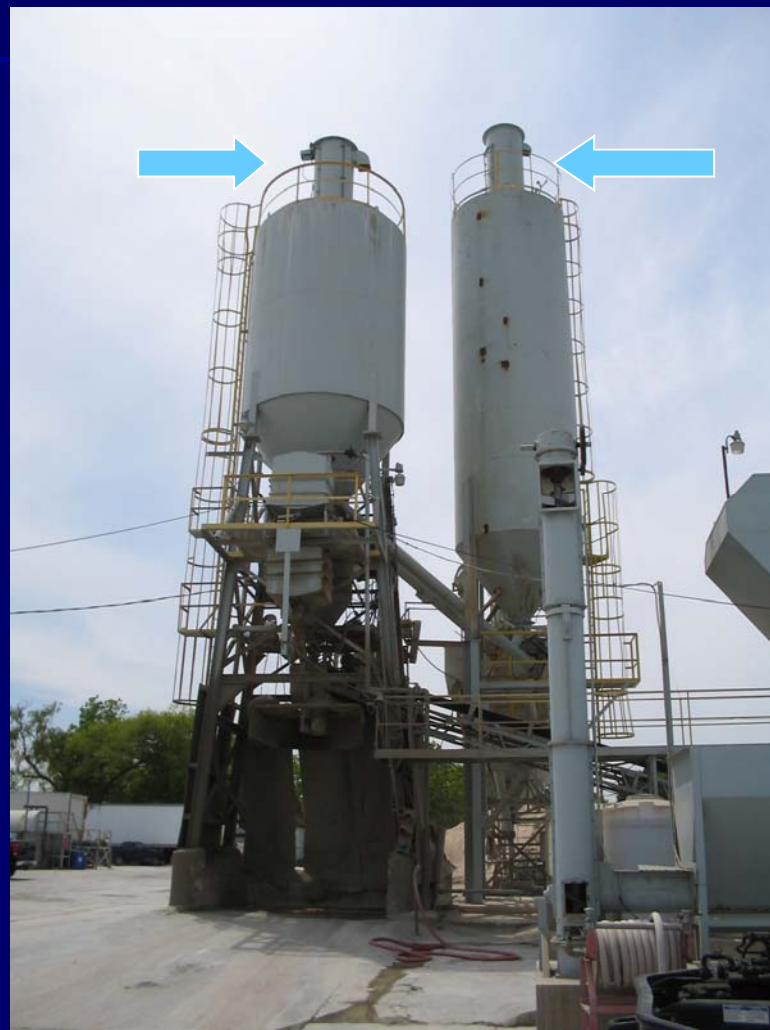
Baghouses on Cement/Fly Ash Silos
