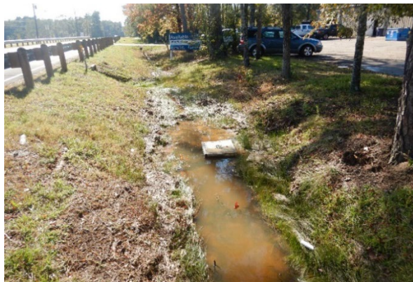
Figure 14 Water retention in ditches
