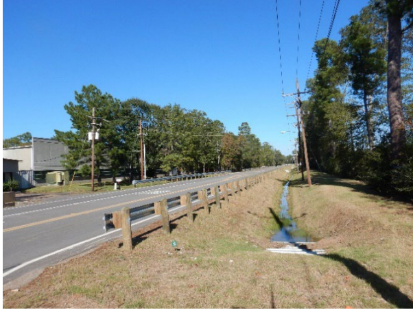
Figure 10 Guard Rails and Unpaved Shoulders on Airport Rd
