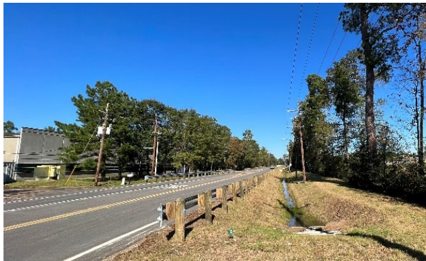
Figure 13 Unpaved Shoulder and Guard Rails between E Dallas St and Venetian Pines. Dr
