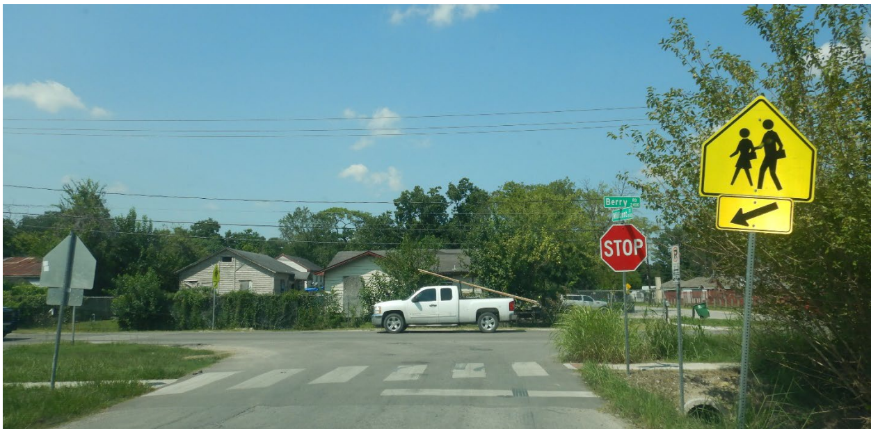
Figure 6. Existing conditions on Berry Road
