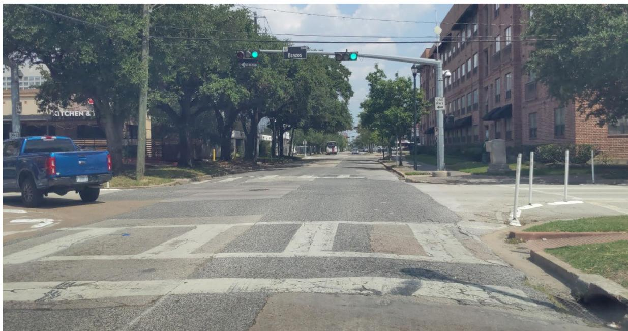
**Figure 28.** Existing pavement on Webster Street is in poor condition
