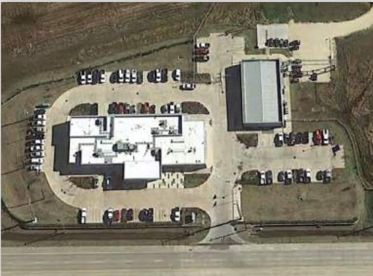
Oneok Partners 12606 TX-146 Aerial Source: Google Earth
