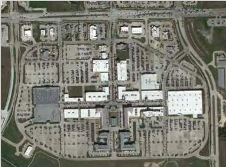
Pearland Town Center Aerial Source: Google Earth
