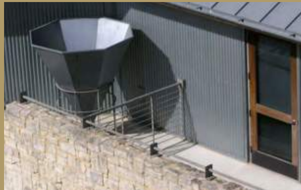
Building roofs are designed to capture and direct rainwater to collection systems on the ground. Source: Lady Bird Johnson Wildflower Center. Austin, TX
