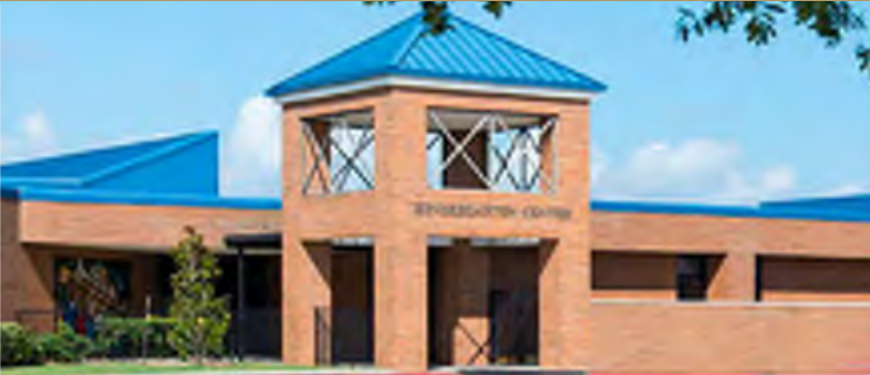
BARBERS HILL KINDERGARTEN CENTER (PRE-K/K) 9696 EAGLE DRIVE
