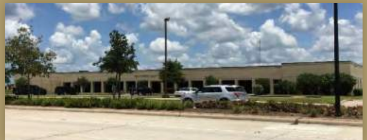
WEST CHAMBERS COUNTY (10616 EAGLE DRIVE)
