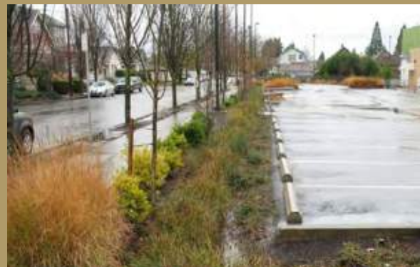
Vegetated swales clean storm water runoff from parking lots and allow it to infiltrate the earth.
