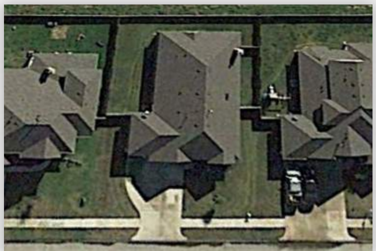
11826 Eagle Ridge Drive in Eagle Point Estate Subdivision Aerial Source: Google Earth
