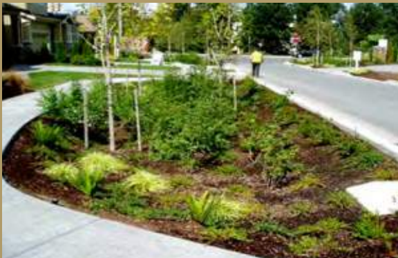
A rain garden is a shallow, constructed depression designed to receive runoff from hard surfaces and planted with deep-rooted native plants.
